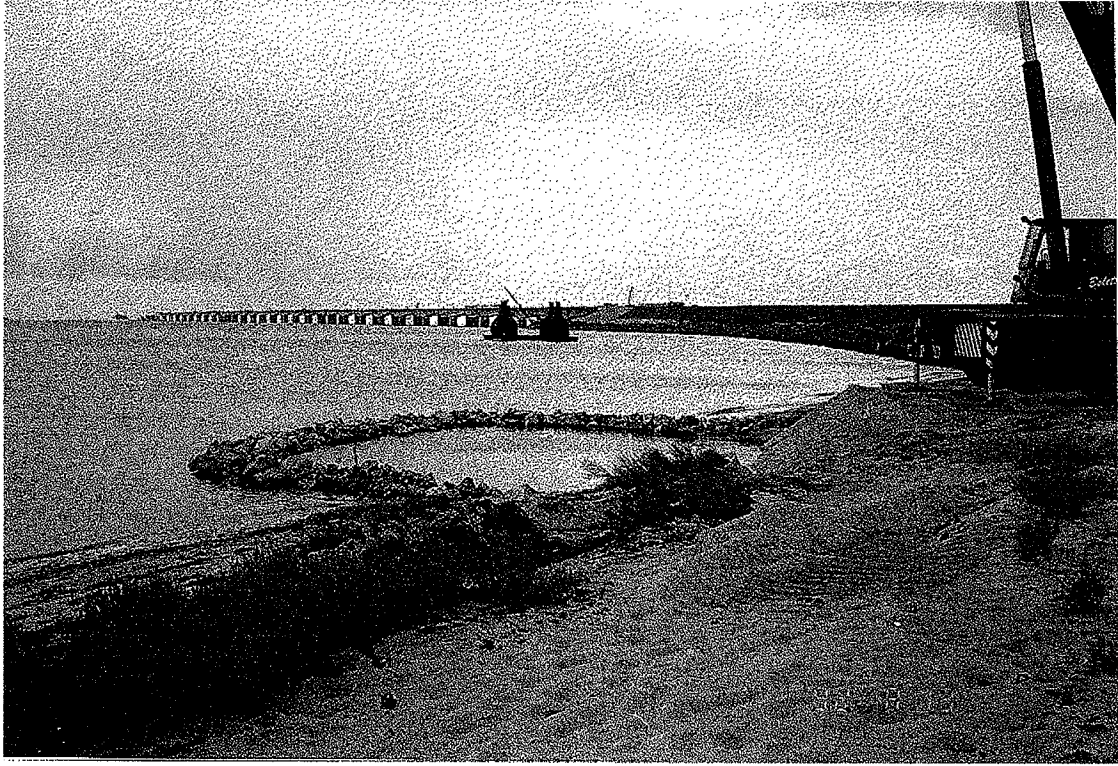
Storebæltsforbindelsens exposure site at Knudshoved. Erosion protection of stones 5-300 kg. August 1992.
