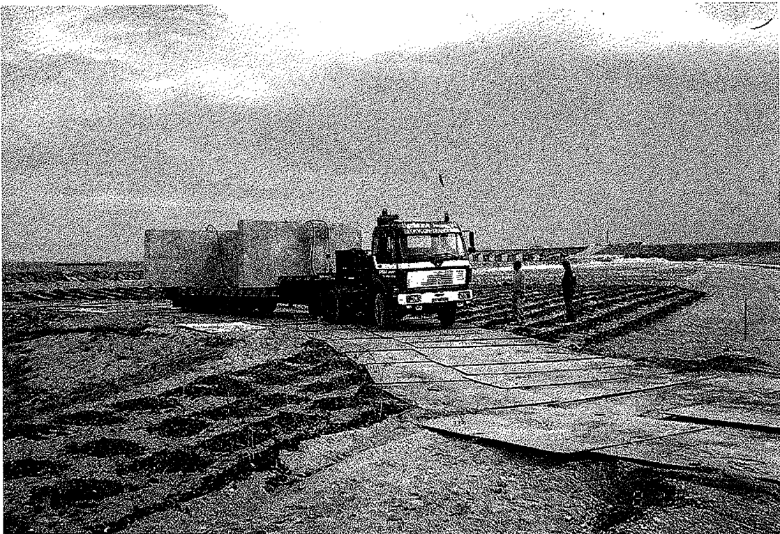
Transport of the approx. 37 ton test element.
