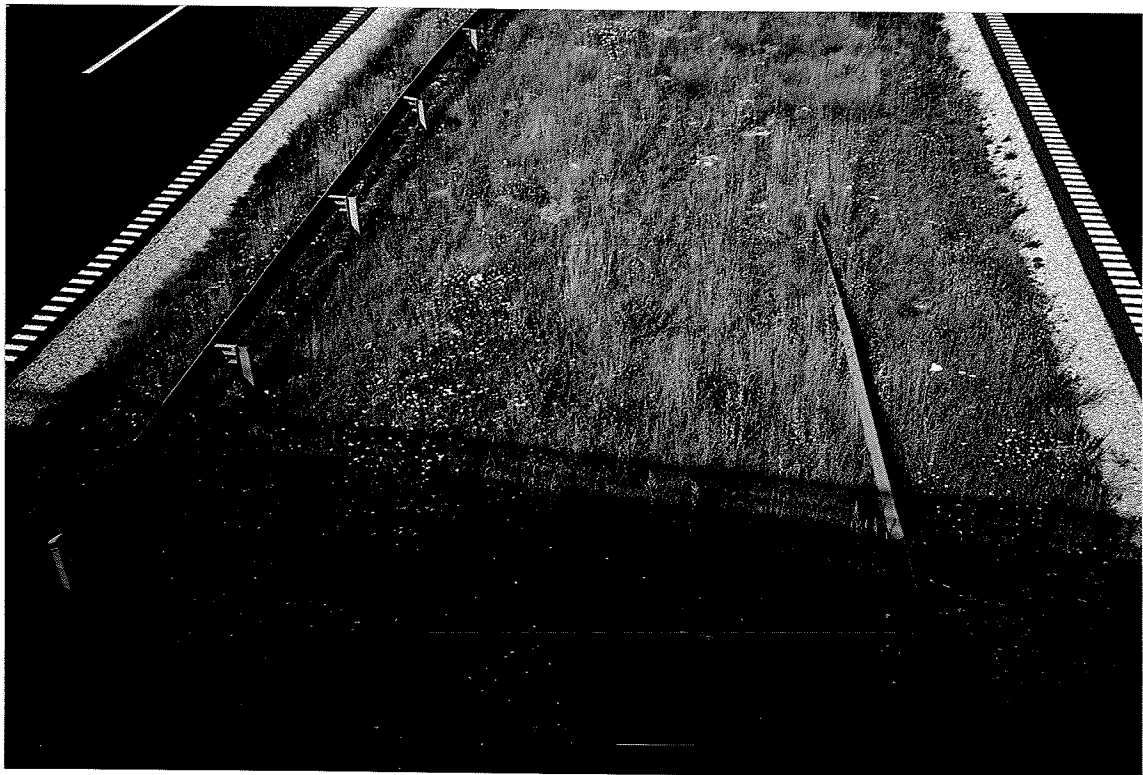
The central reservation is approx. 9 m wide.
