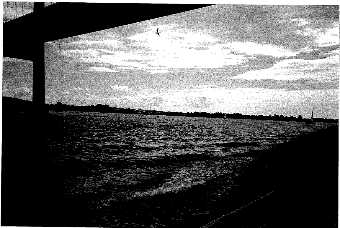
New Little Belt Bridge. Sea bed gradient approx. 1:4.
