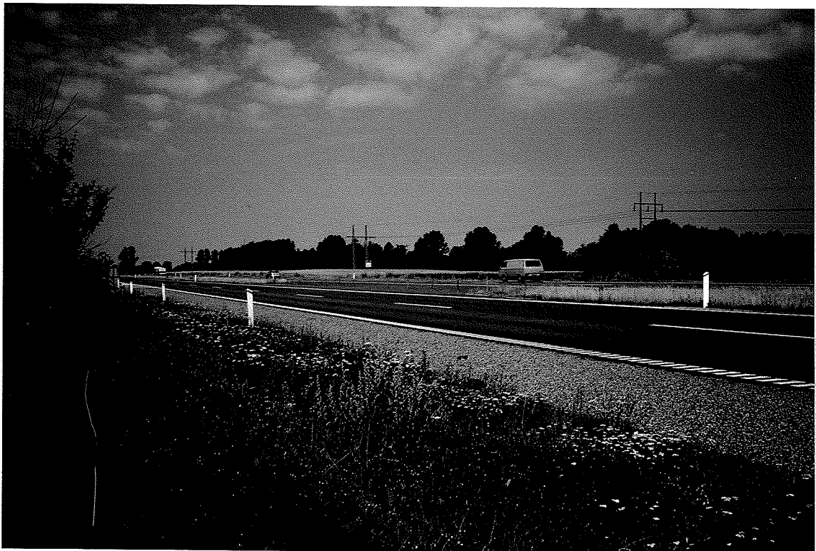
The central reservation at Kongsted is the same width (approx. 9 m) as the whole stretch Ringsted-Kongsted.
