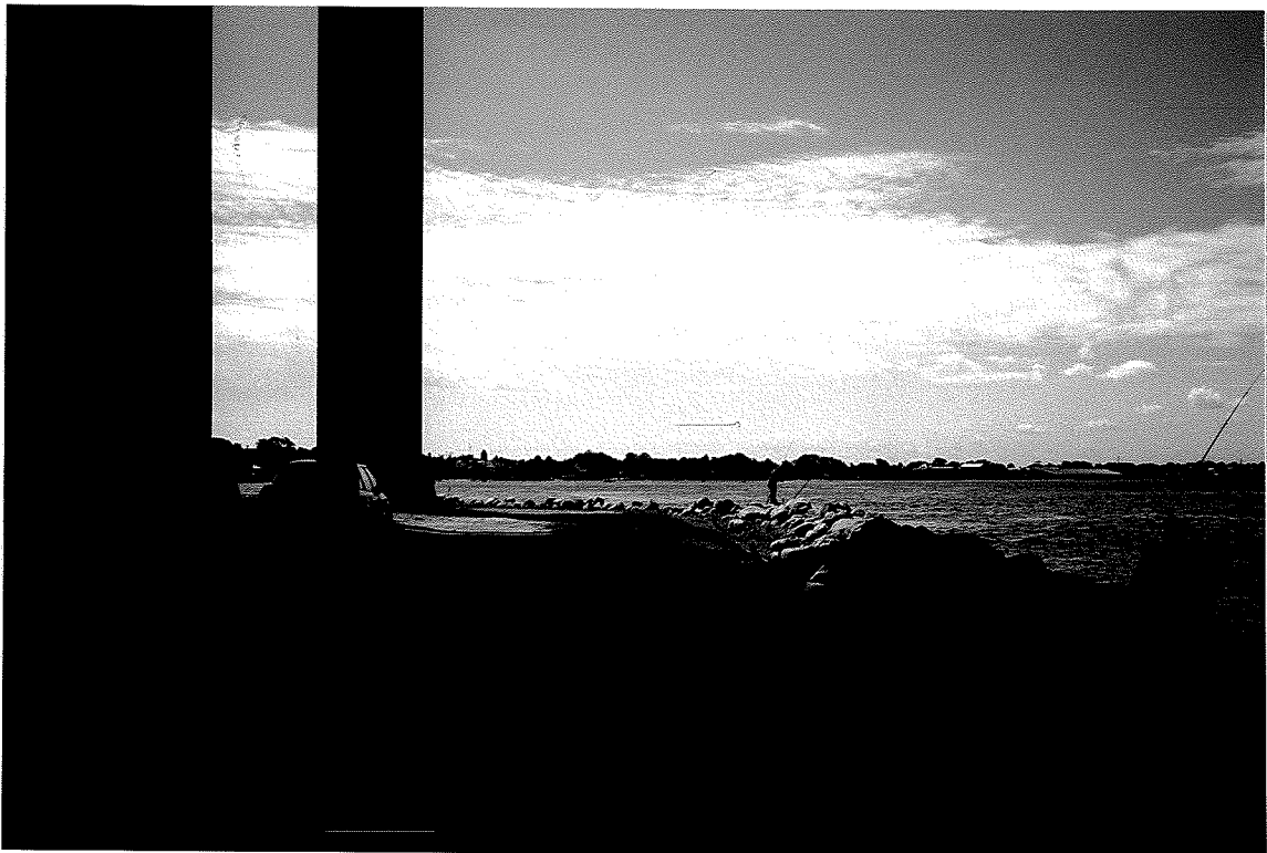
Popular place for fishing. Extensive erosion protection. Relatively large distance from gravel road.
