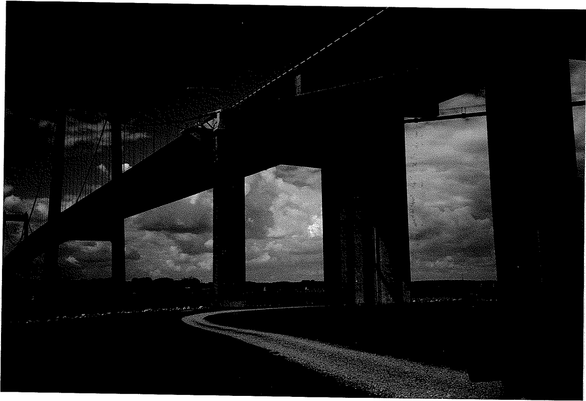
New Little Belt Bridge, Fyn side. Good accessibility on public gravel road.
