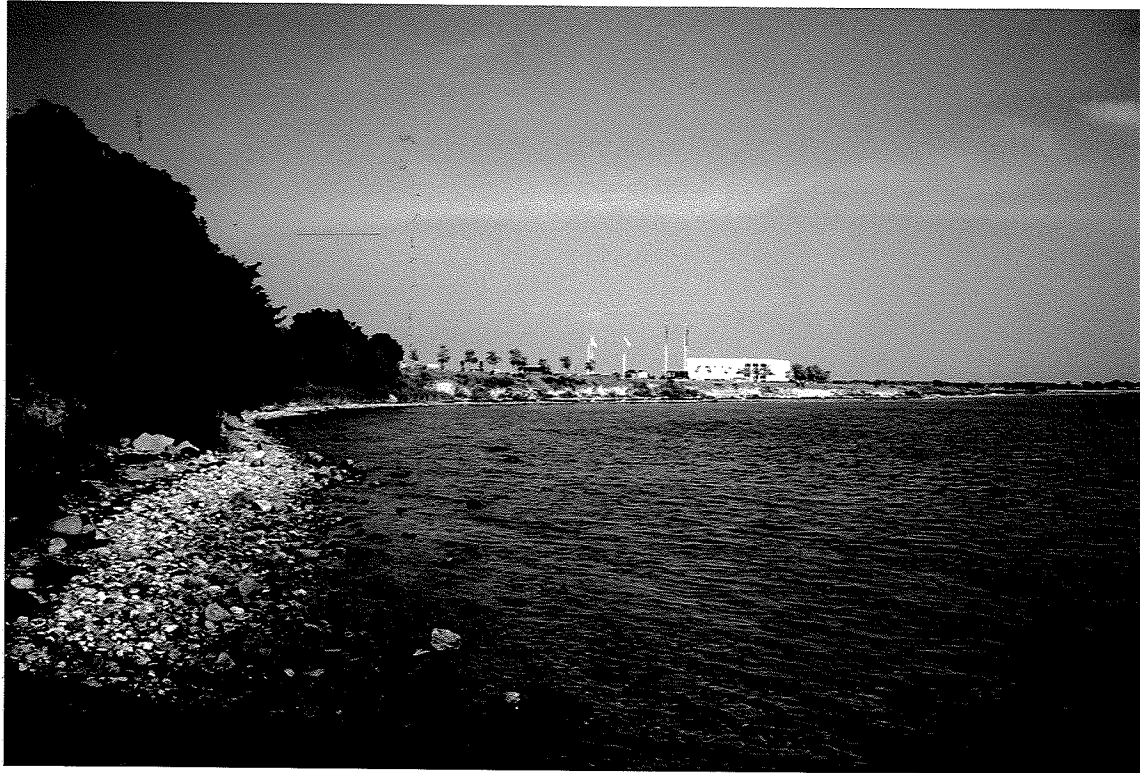
Farø east of the abutment of the cable-stayed bridge. Cafeteria and exhibition buildings.
