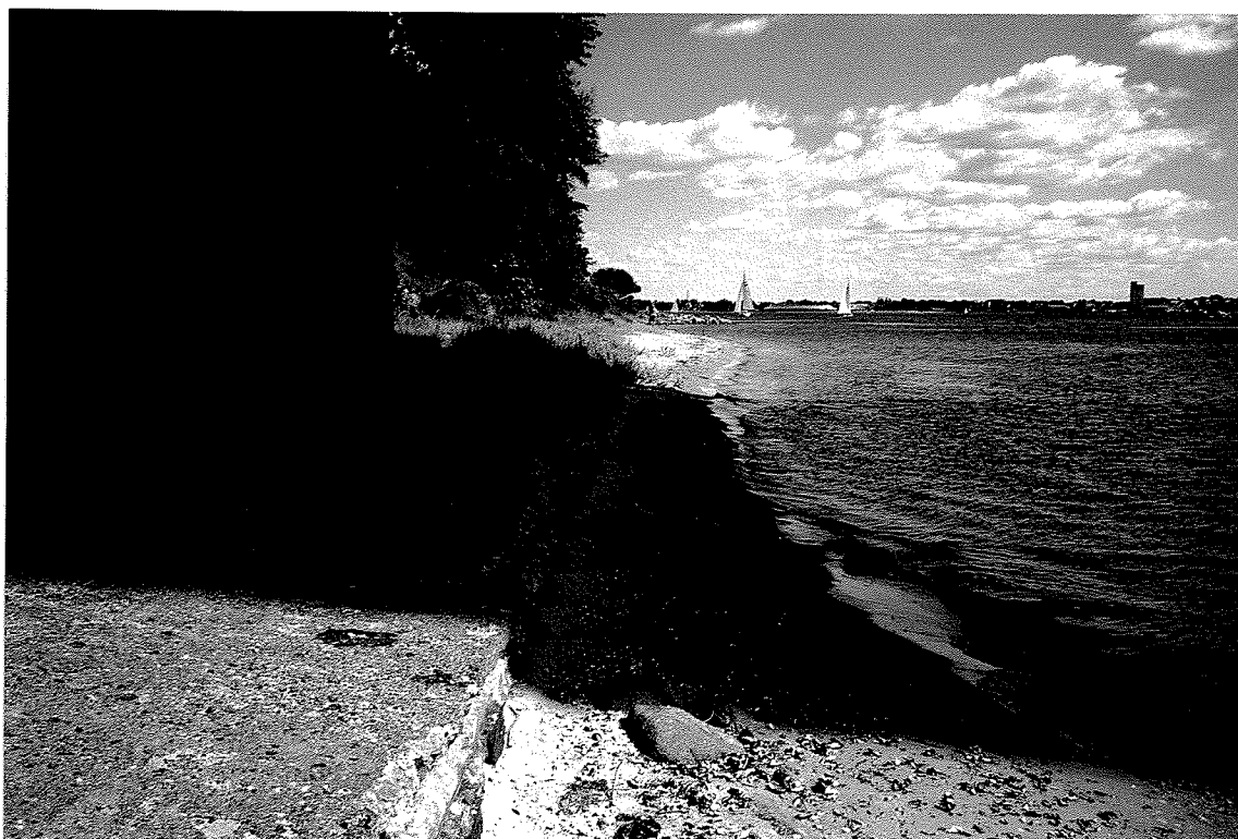
Old Little Belt Bridge, Snoghøj, Jylland. Foundation slab.
