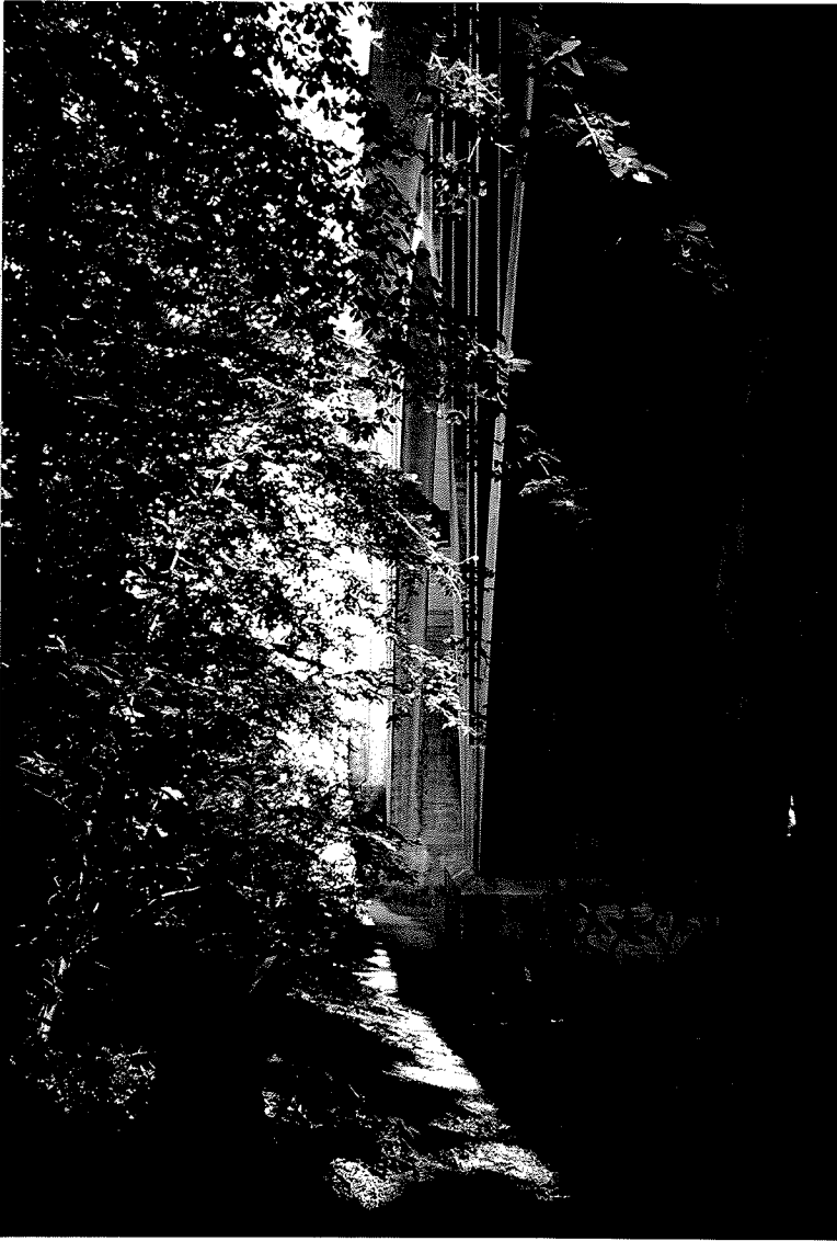
Old Little Belt Bridge, Kongebro, Fyn. No access by truck.
