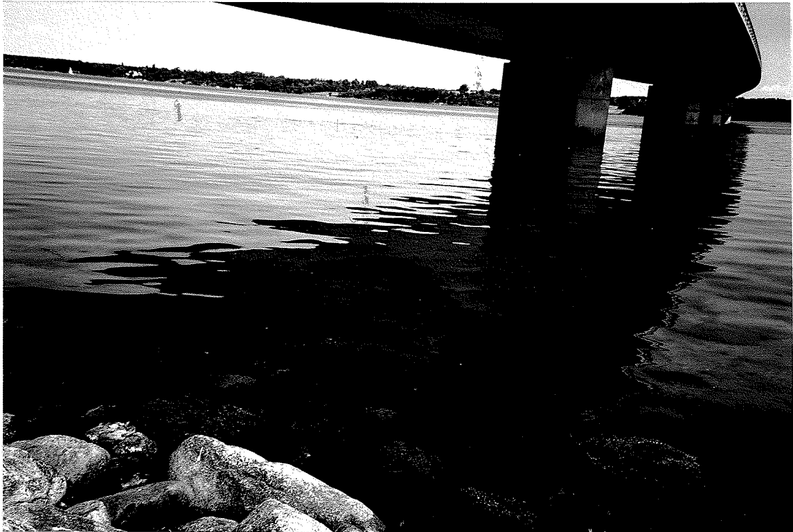
Farø north. Low water level approx. 1 m at first pier.
