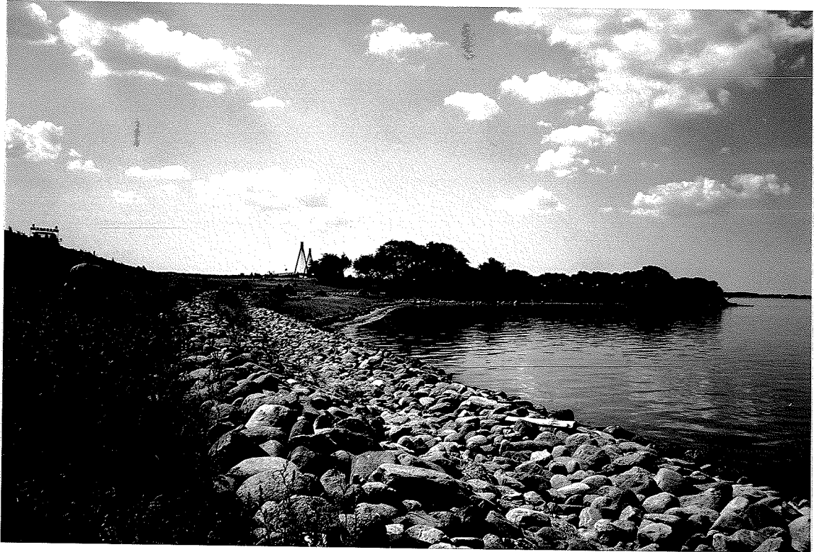
Farø northwest. Area with shallow water. Poor accessibility from land and sea.
