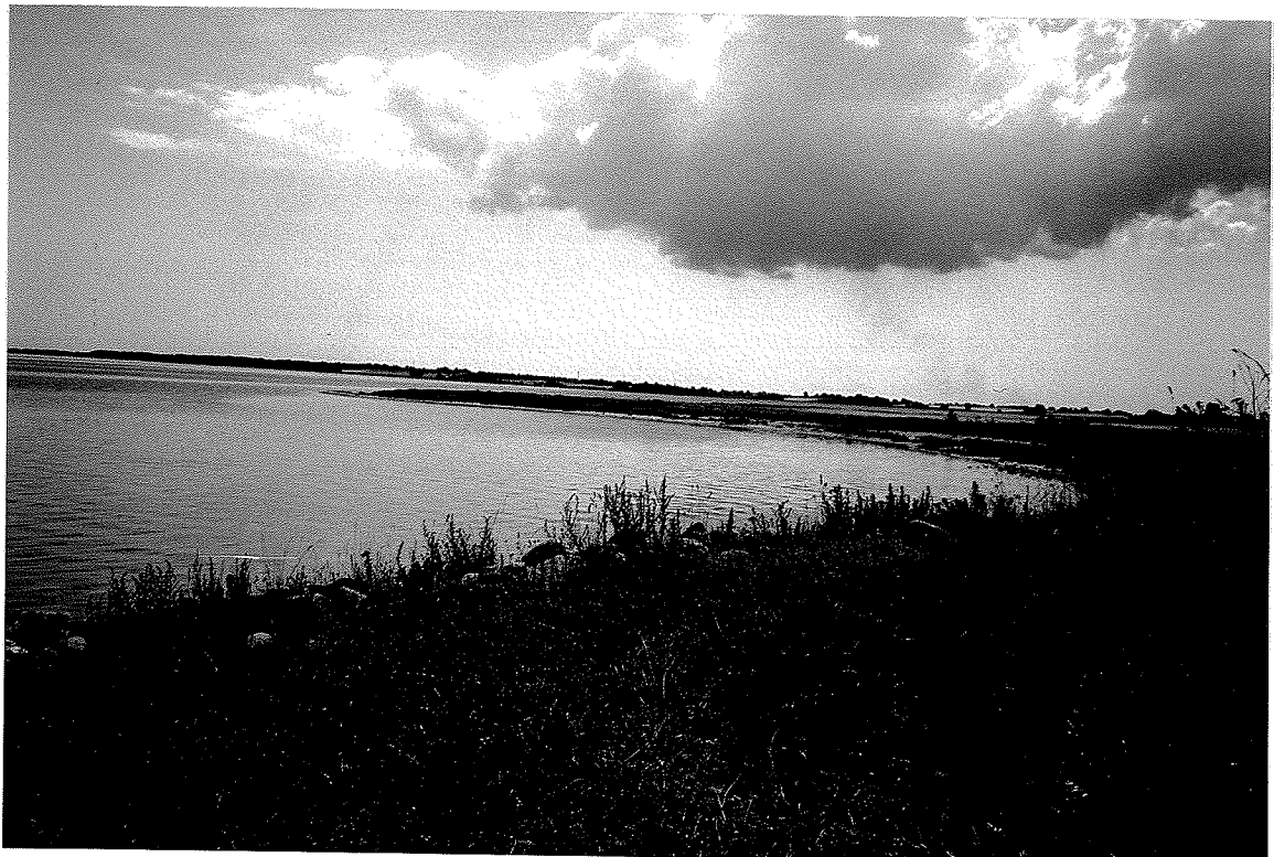
Farø northeast. Erosion of fill-area east of the bridge.
