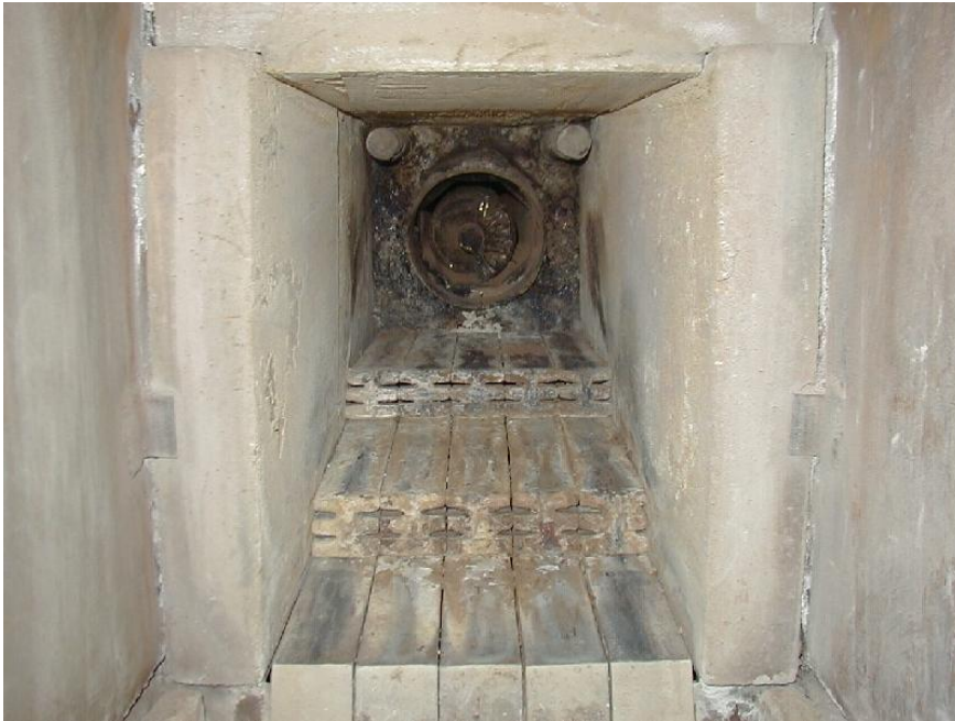
Picture 8-6. Clean combustion chamber.
