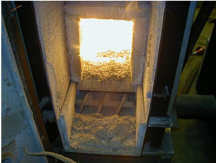
Picture 8-22. The picture was taken shortly before shut down. A small quantity of slag was found in the ash, but it was crumbly and therefore easily removed by the ash screw. The combustion chamber was slightly fouled.
