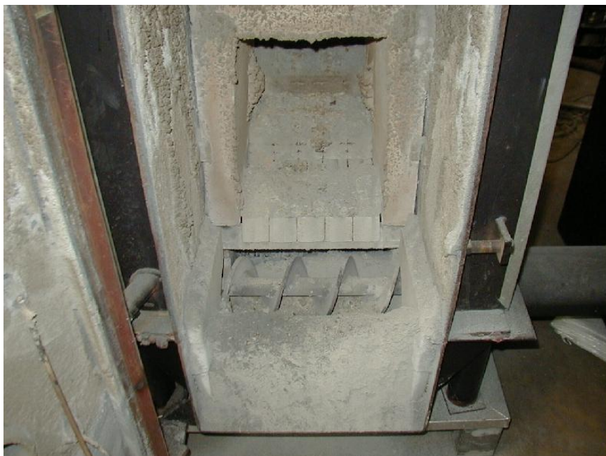
Picture 8-16. The picture was taken shortly after shut down. There was a large quantity of ash in the ash box, but no slag was found because the ash screw had been able to remove the slag continuously. Therefore, the quantity shown in the picture was constant. The combustion chamber was very heavily fouled and fixed slag was found both at the refractory and at the air nozzles.
