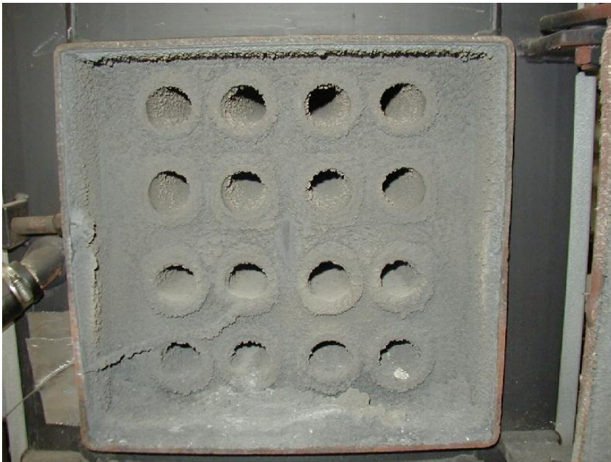
Picture 8-9. The worst case of fouling after 65 hours. From R4.
