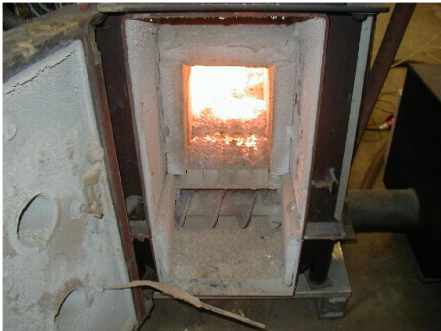
Picture 8-20. The picture was taken shortly before shut down. A large quantity of ash was found in the ash box, but no slag was found. The combustion chamber was slightly fouled.
