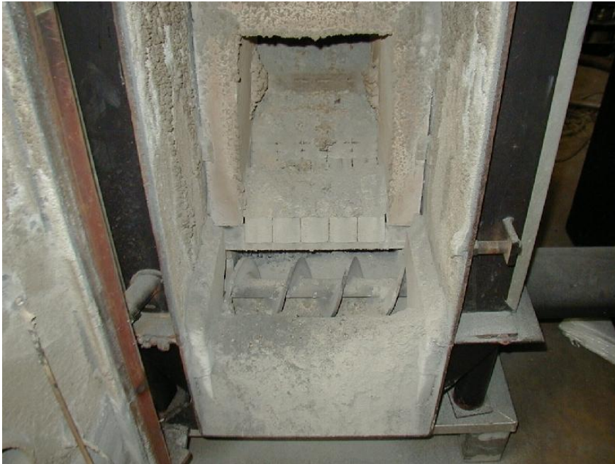
Picture 8-4. Typical ash quantity in the boiler when there is no slag. Ash from R4.
