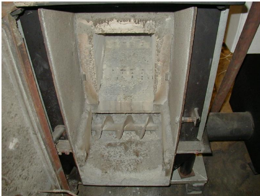
Picture 8-18. The picture was taken shortly after shut down. There was a large quantity of ash in the ash box, but no slag was found in the ash. The combustion chamber was slightly fouled.
