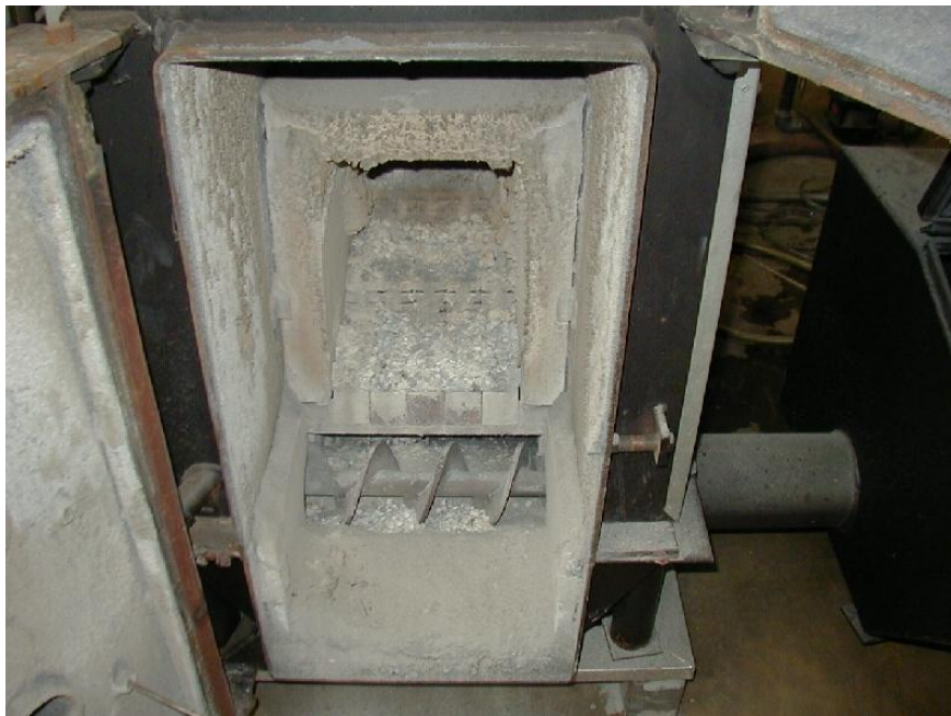
Picture 8-17. The picture was taken shortly after shut down. There was a large quantity of ash in the ash box, but no slag was found in the ash. The combustion chamber was very heavily fouled and fixed slag was found both at the refractory and at the air nozzles in spite of the fact that the test duration was relatively short.
