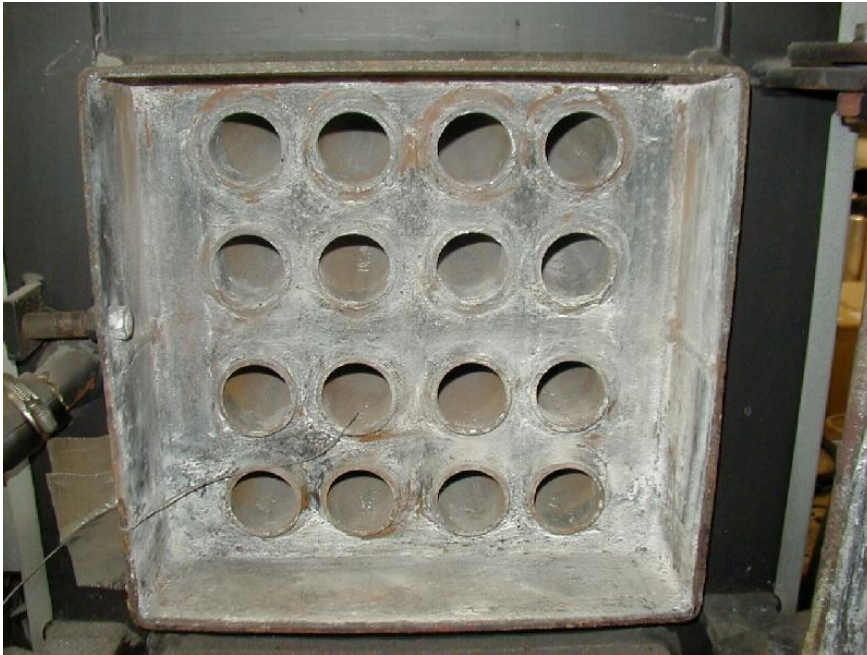
Picture 8-8. Clean flue gas tubes before the test.
