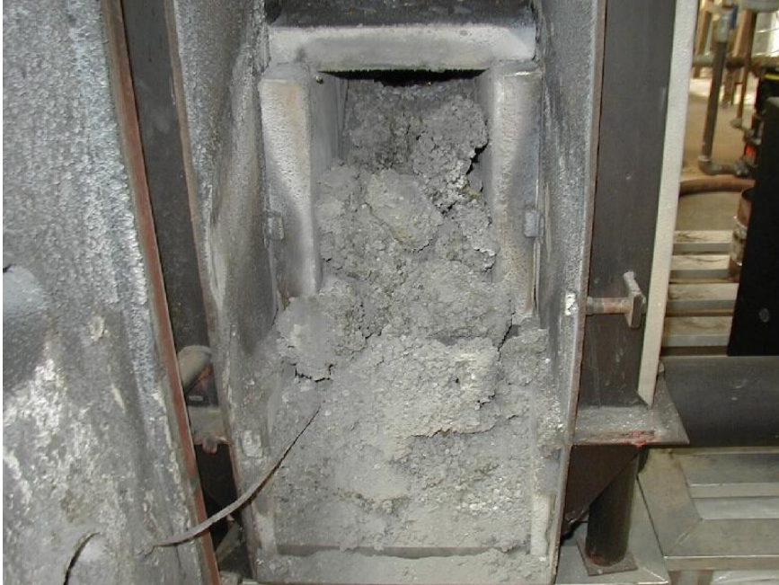
Picture 8-2. Typical slag formation. Slag from R3.
