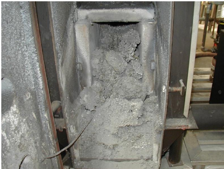
Picture 8-15. The picture was taken shortly after shut down. The combustion chamber was completely filled with slag. In addition, the combustion chamber was heavily fouled.
