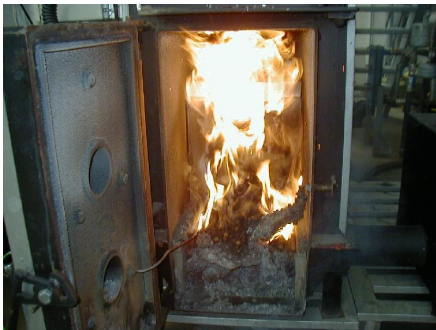
Picture 8-13. The picture was taken shortly before shut down. There was a lot of slag which the ash screw had not been able to remove. This made the fuel accumulate in the combustion chamber. When the boiler door was opened, some of the slag fell out and the accumulated fuel was ignited.
