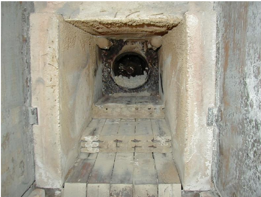
Picture 8-7. Typical picture of fixed slag. The fixed slag is primarily concentrated at the primary air nozzle. From R10.
