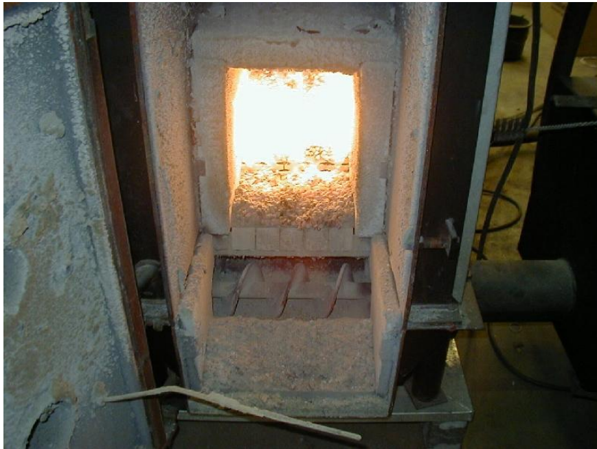
Picture 8-23. The picture was taken shortly before shut down. A large quantity of ash was found in the ash box, but no slag was found in the ash. The combustion chamber was slightly fouled.
