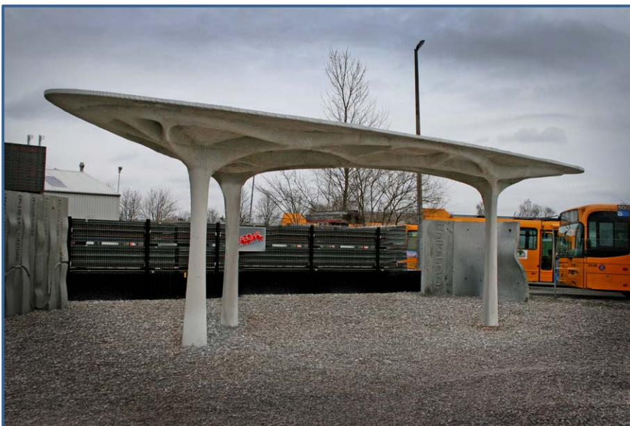
Fig. 17: Concrete pavilion from 2010 made in connection to the research project Unique Concrete Structures. The formwork was created using the robot cell at Danish Technological Institute.
