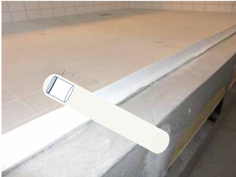
Figur 8: Sensorns placering i betongplatta
