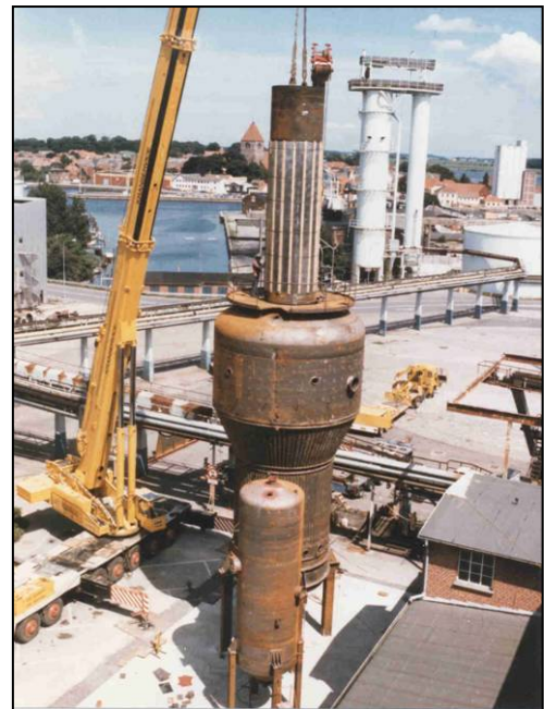
Figure 7. Construction of the prototype.
