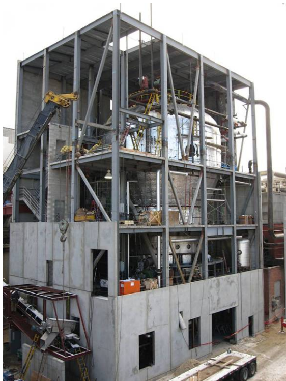
Figure 19. The drier in Nampa, Idaho under erection.
