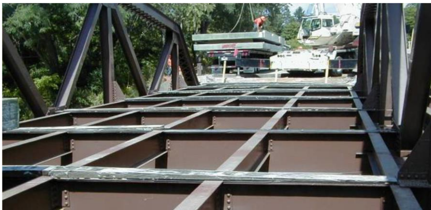
Figur 2.3-3: Restaurering af broen "Route 367 over Bentley Creek" i Wellsburg, New York.
