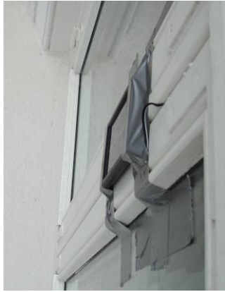
Figure 21 Solar Cell on window frame
