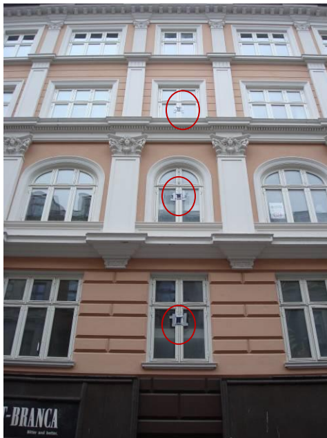
Figure 24 Solar Cells on the facade, Oehlenschlägersgade 49
