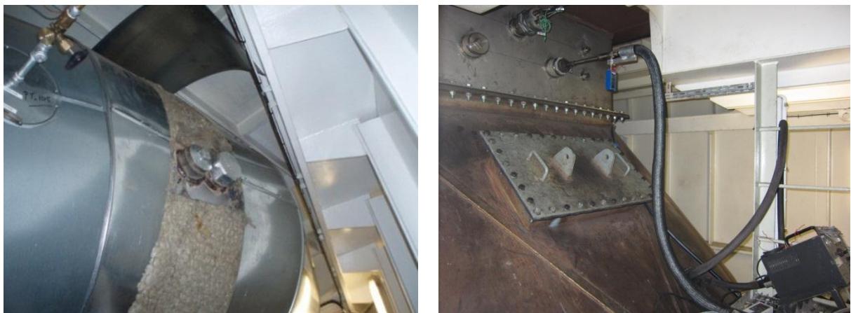
Figure 3: Probe socket connectors. The pictures show the sample outlets before (left) and after (right) the scrubber.
