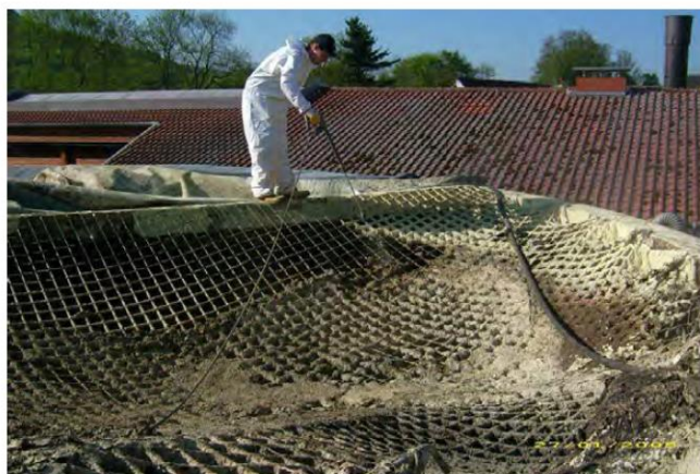
Figure 2: Sulfur precipitation in a digester (Beil, 2010)
