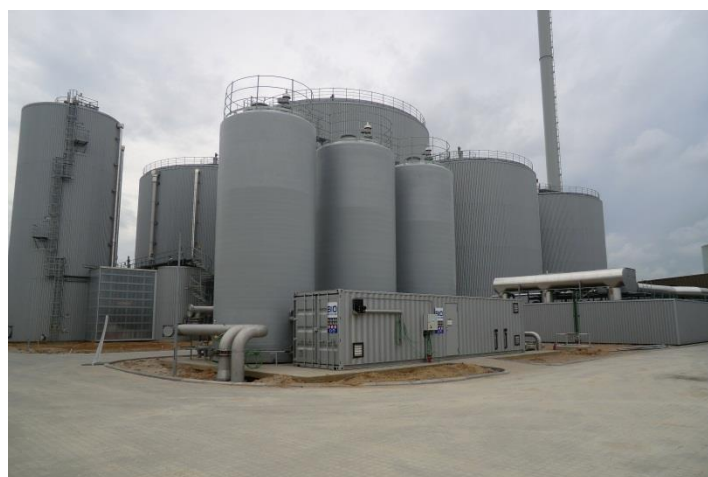
Figure 8: BioGasclean Måbjerg plant
