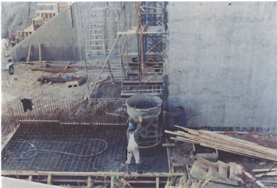
Figure 17. The concrete was placed in the mould by use of a buggy
