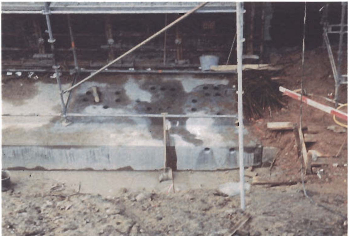
Figure 20. The foundation after some of the samples had been taken.
