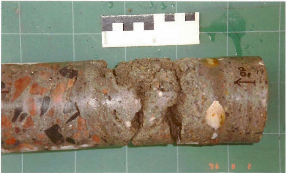
Figure 11: Bottom of the shotcrete repair of a bridge from 1987 (Bridge 3). The repair is very porous and the middle section has not been filled at all. The craftman has not been able to fill the repair while spraying from below which is the worst angle to use the shotcrete technic.
