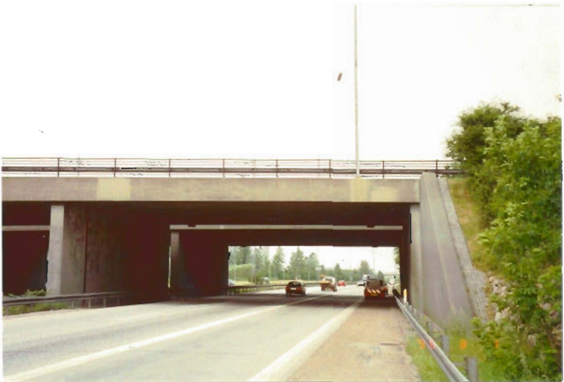
Figure 8: Bridge 4 was built in 1978. The two repairs which were inspected were holes from bad compaction on the outside of the edgebeam. The defects were repaired with shotcrete.
