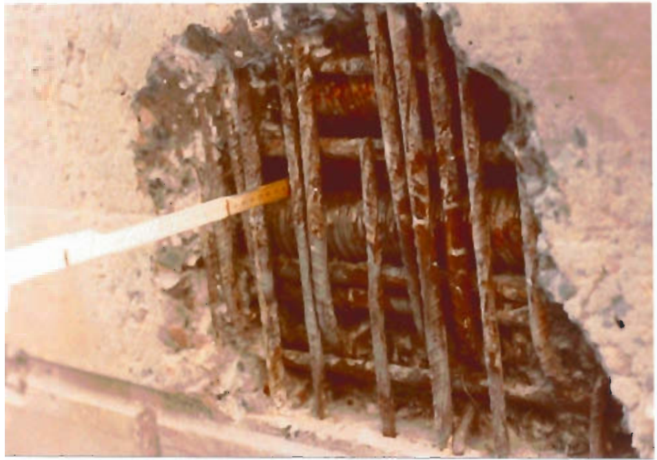
Figure 7: Underside of bridge 3 box girders after form stripping before repair.
