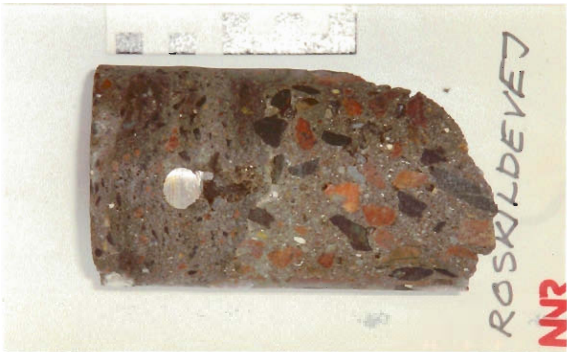
Figure 12: Shotcrete repair of the sidebeam of a bridge from 1978 (Bridge 4). There is a hole in the shotcrete behind the reinforcement. The craftman has not been able to fill the hole while spraying.
