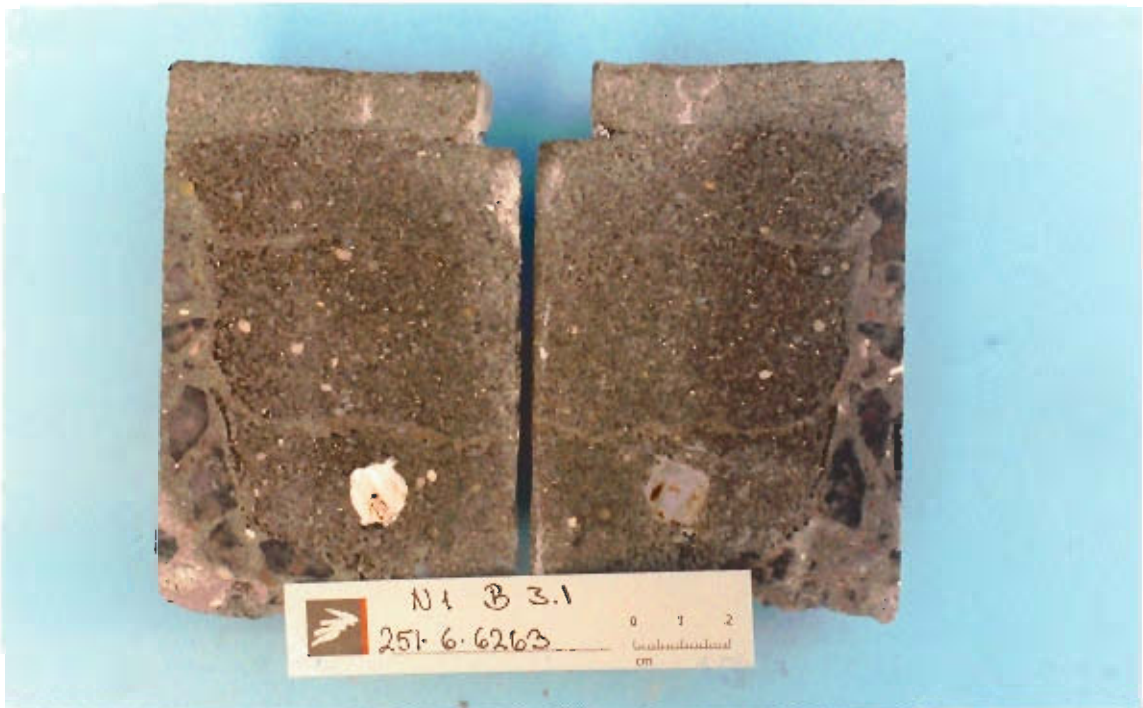
Figure 14: Repair with mortar on the inner side of the edge beam of bridge from 1996 (Bridge 2). The mortar is porous due to bad compaction and mixing and there is a weak section near the bottom part of the repair.
