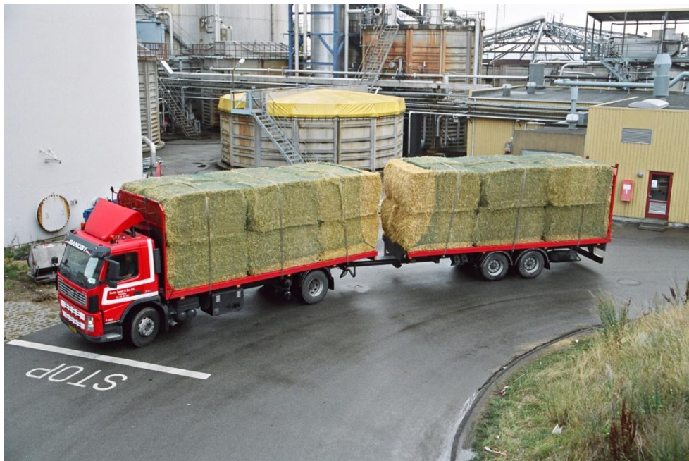
A truck load of straw arrives at the Power Plant
