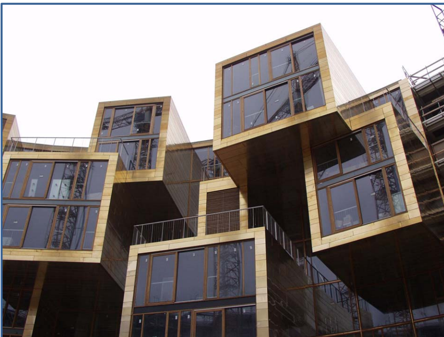
Fig. 3: Tietgen Collegium, Copenhagen. The circular main building has 45 hanging concrete boxes in two stories, which contain kitchens and other common facilities. The largest boxes have a free span of 8 m and weigh 250 tons. Cowi, the consultant company, solved this structural challenge by using innovative solutions and "free forward construction". It is a construction method that normally is applied for building bridges. The method has no need for scaffoldings and the result is a significant saving in time and money.
