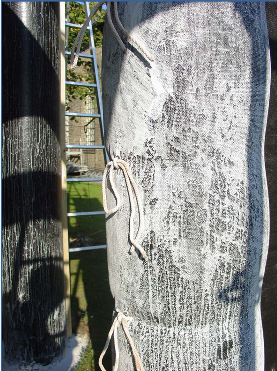
Fig. 6: Textile formwork used for the casting of a concrete column.
