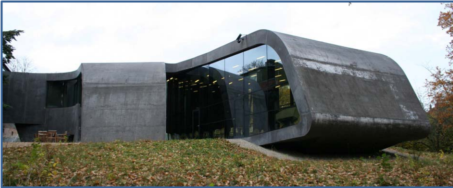
Fig. 2: The extension of the Ordrupgaard Museum in Copenhagen. Complex shape cast in self-compacting concrete.
