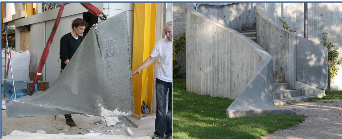
Fig. 27: The finished concrete elements.
