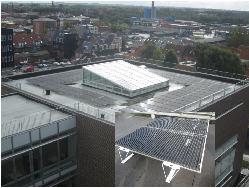
Installation with the unique tubular Solyndra PV modules (CIS). Skive Library, 18 September 2012
