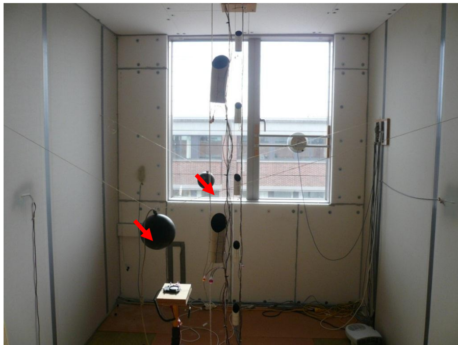
Figure 4.3 Globe temperature sensors in one of the test rooms.
