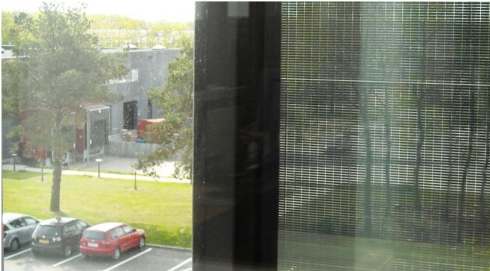
Figure 2.2 a-Si TFPV module used as solar shading device in a moving solar shutter. The picture is taken as the device is closing, whereby the transparency of the device is shown and can be compared with the view without the shutter (EnergiMidt, Silkeborg).
