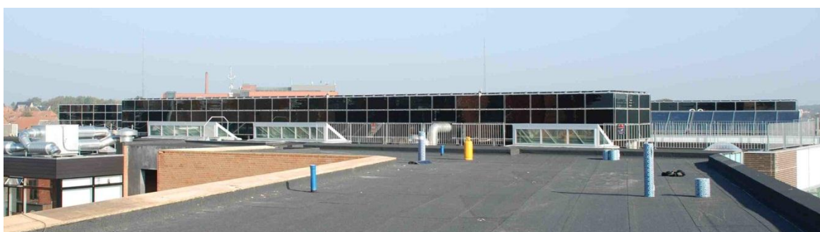
Figure 2.1 CdTe TFPV modules utilized to covered technical installation at the rooftop of Skive City Hall.
