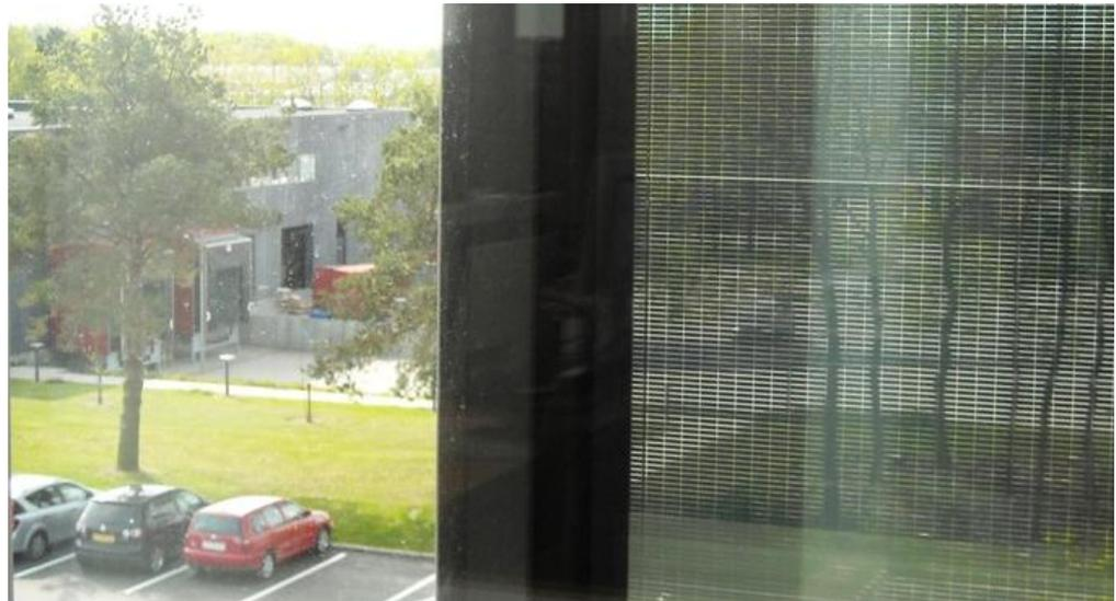
a-Si TFPV module used as solar shading device in a moving solar shutter. The picture is taking as the device is closing, whereby the transparency of the device is shown and can be compared with the view without the shutter (EnergiMidt, Silkeborg).
