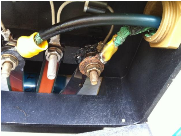
Corrosion of terminals and heat damage of junction box on module E1.
