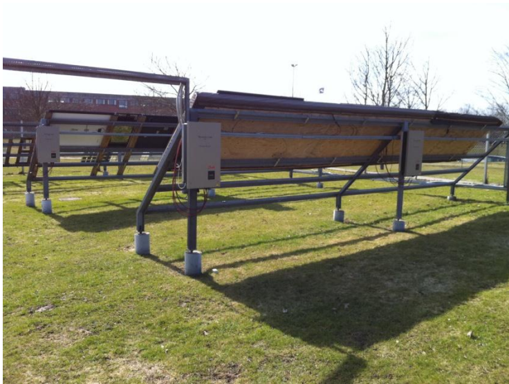
The two module racks seen from behind.
