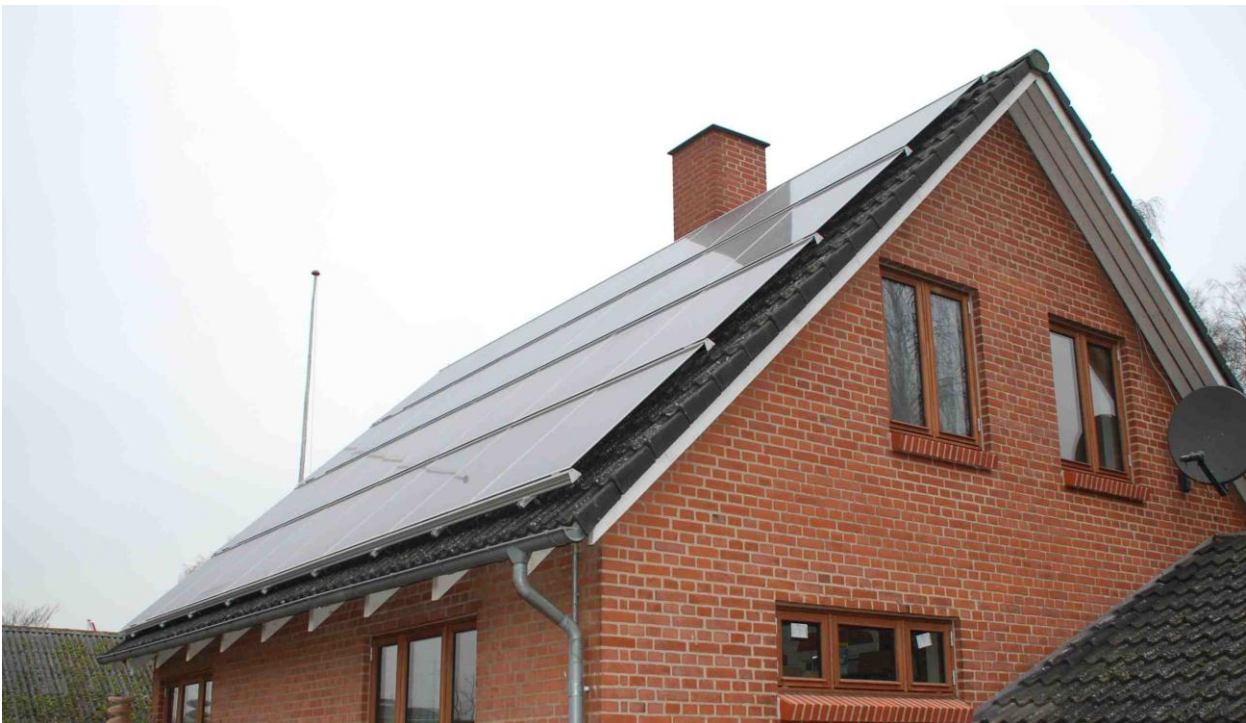
The same a-Si/ \mu c-Si TFPV plant from another perspective.
