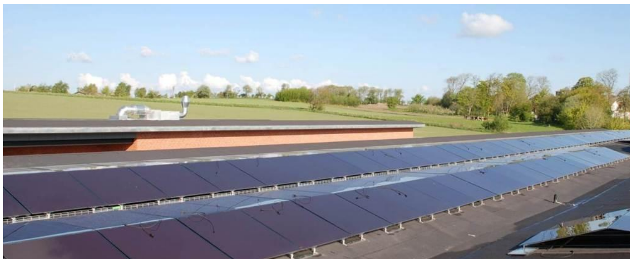
a-Si thinfilm modules installed at Plejecenter Marinelyst in Skive.
