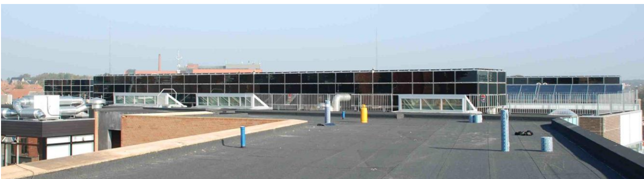
The covered technical installation after completion of the TFPV plant. The ventilation plant visible to the left does not belong to the city hall.
