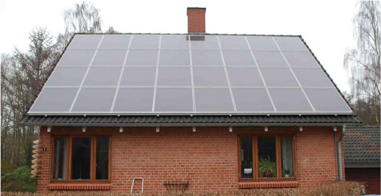
a-Si/ \mu c-Si modules mounted on south facing roof surface.
