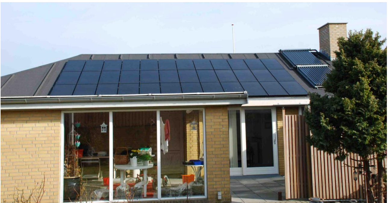
CIGS modules on east facing roof surface. Vacuum solar collectors for hot water production is placed to the right.
