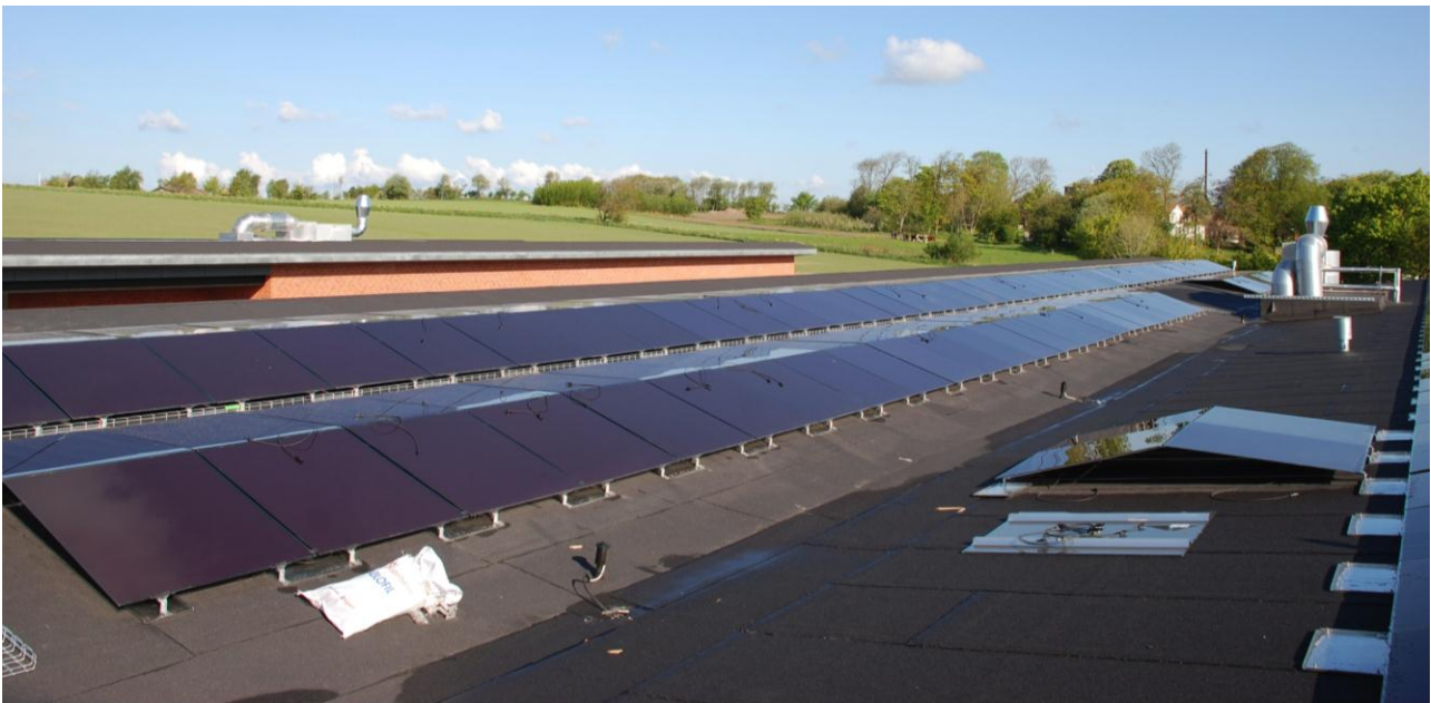
East-west facing a-Si modules placed on Plejecenter Marienlyst.
