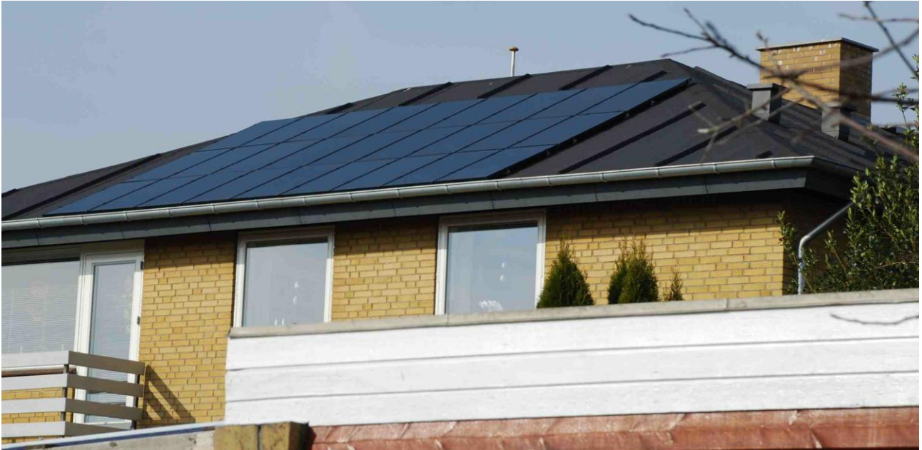
CIGS modules placed on south facing roof surface.
