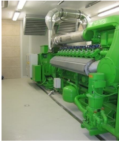
Power generation gas-engine – CHP.
