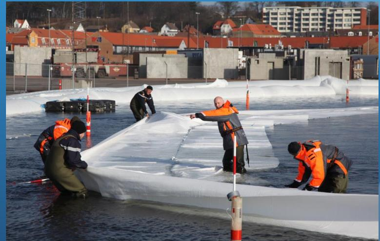
⇒ In 5 hours, 5 men using a vehicle can deploy 1000 meters of flood barrier (80 cm flood water)
