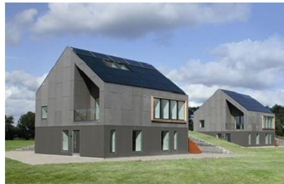
Figure 1: EnergyFlexHouse with PV panels on the roof. Left house: The test house in use. Right house: Identical house occupied by a single family.
