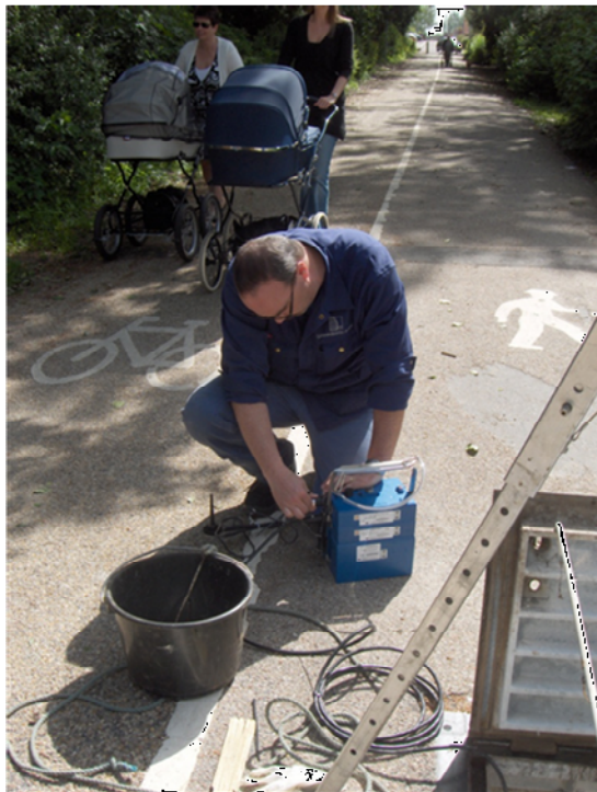
Battery, modem and flow-logger
