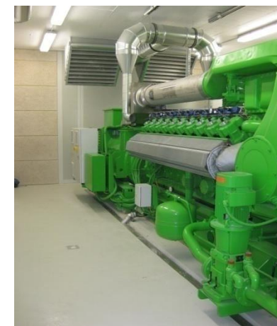
Power generation gas-engine – CHP.
