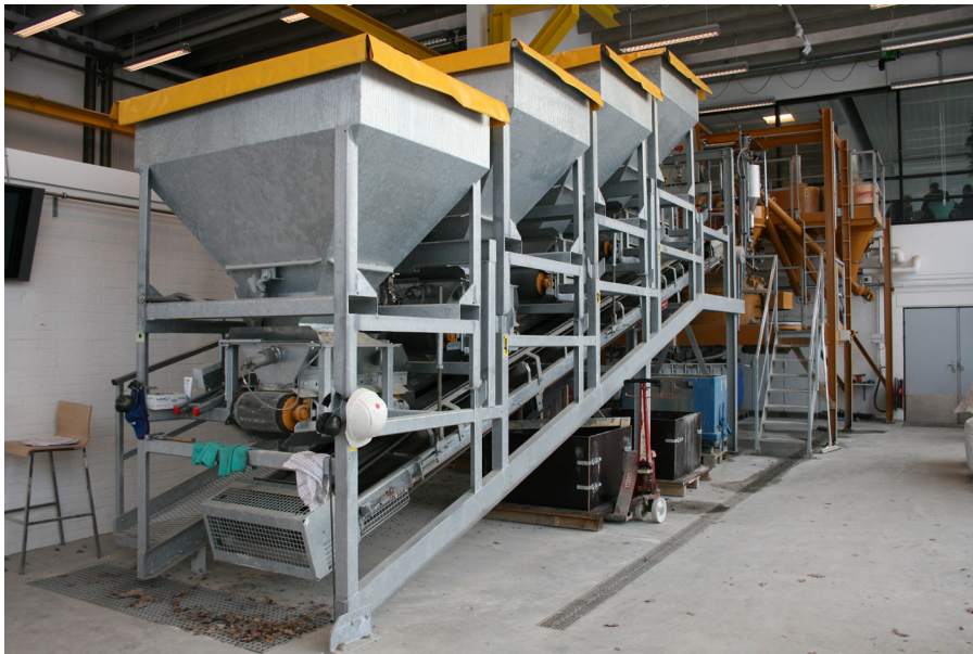
Mixing plant at DTI's Concrete Centre
