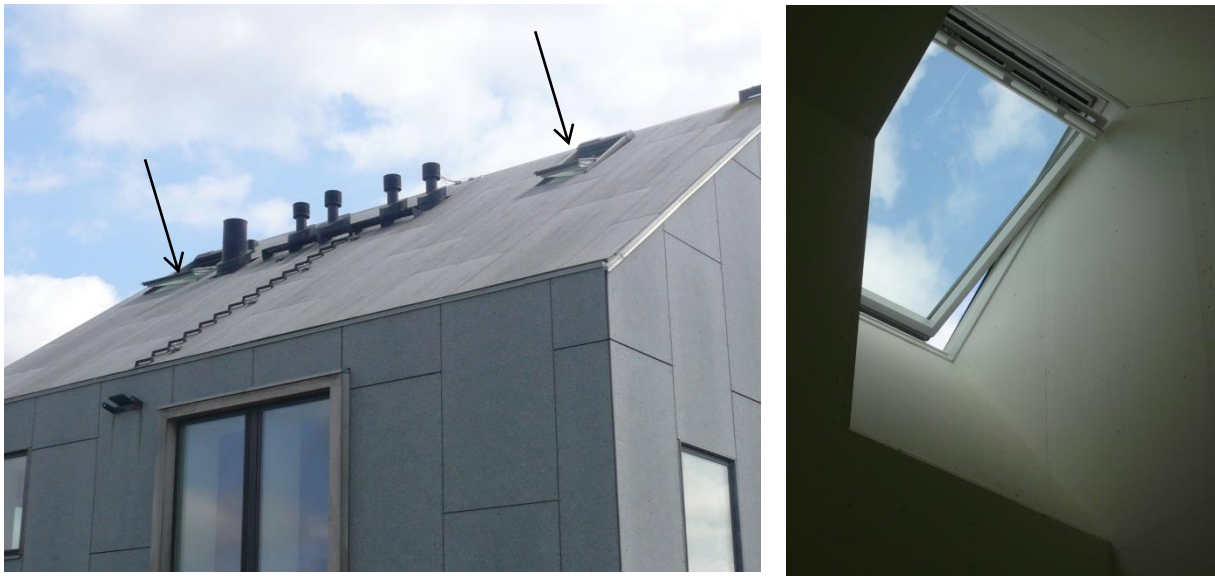
Figure 2.6. The two roof windows seen from the outside and the inside.
