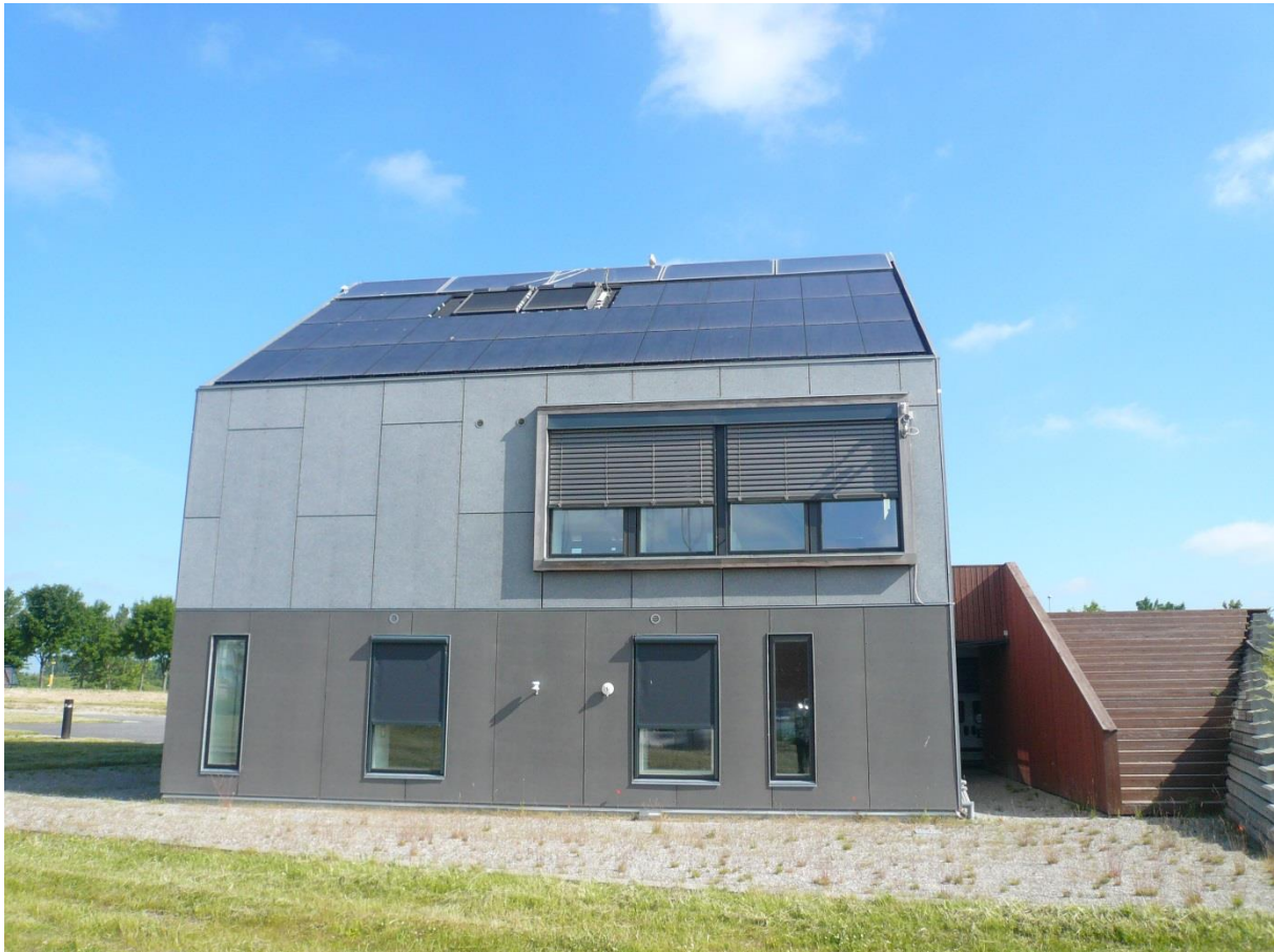
Figure 2.8. The movable solar screening on the south façade and south facing roof.
