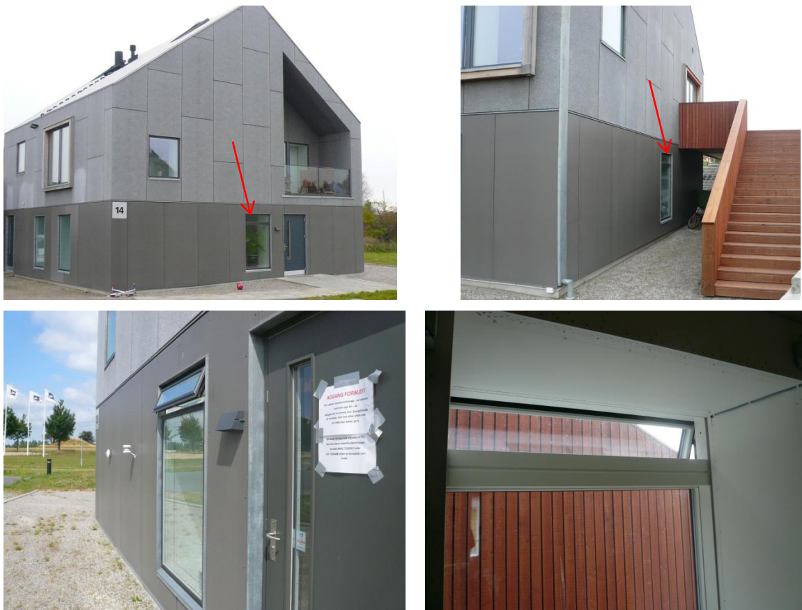
Figure 2.7. The two small operable windows in each end of the aisle.
