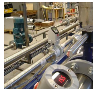
Test of circulation pumps.
