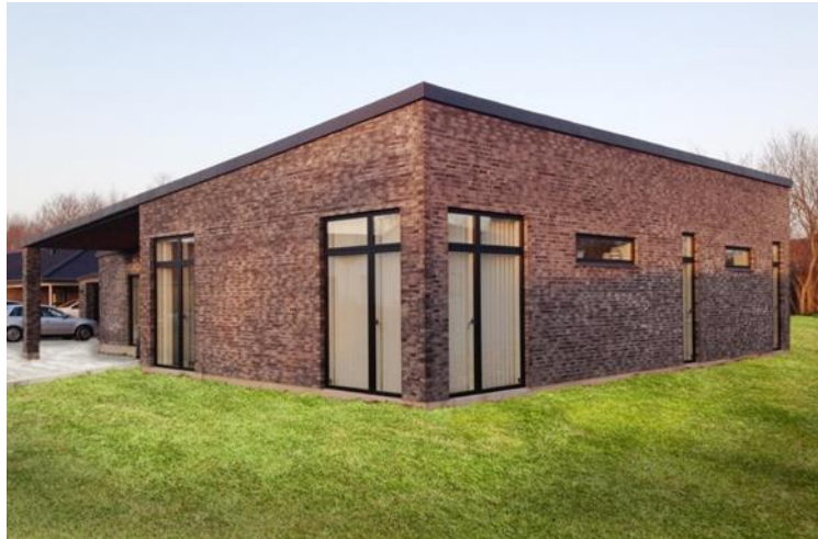
Figure 5.1: Picture of the test house seen from South-West.
