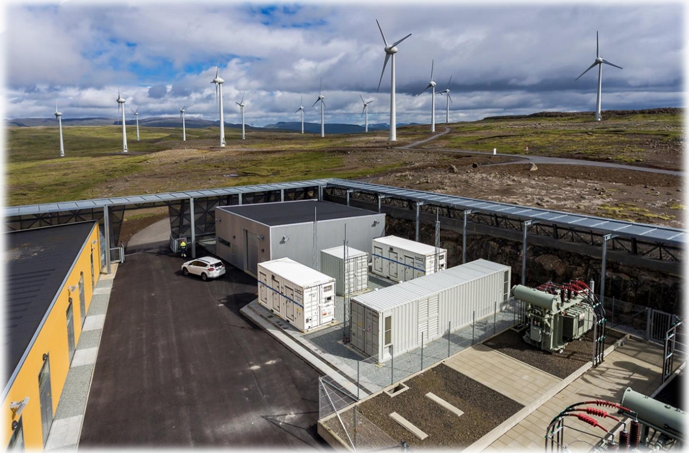
Battery system in Húsahagi, Faroe Islands
