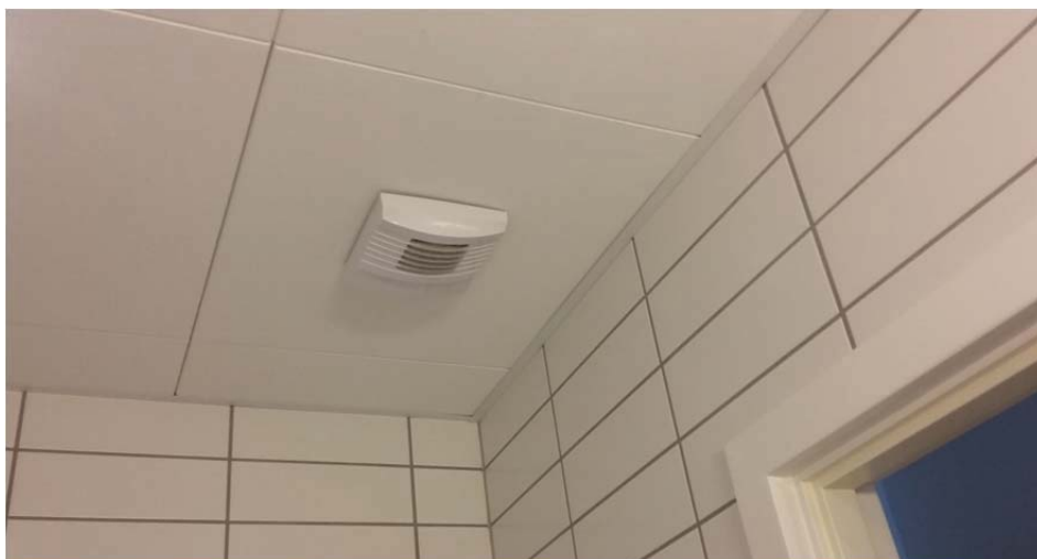
Air extract terminal, example
