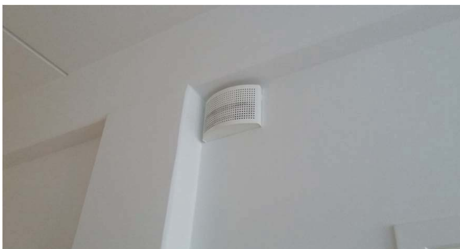
Air supply terminal, example
