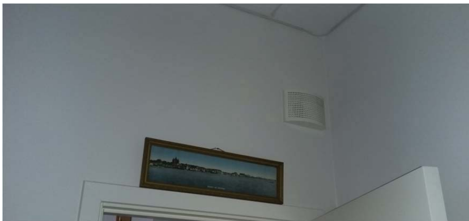
Air supply terminal, example
