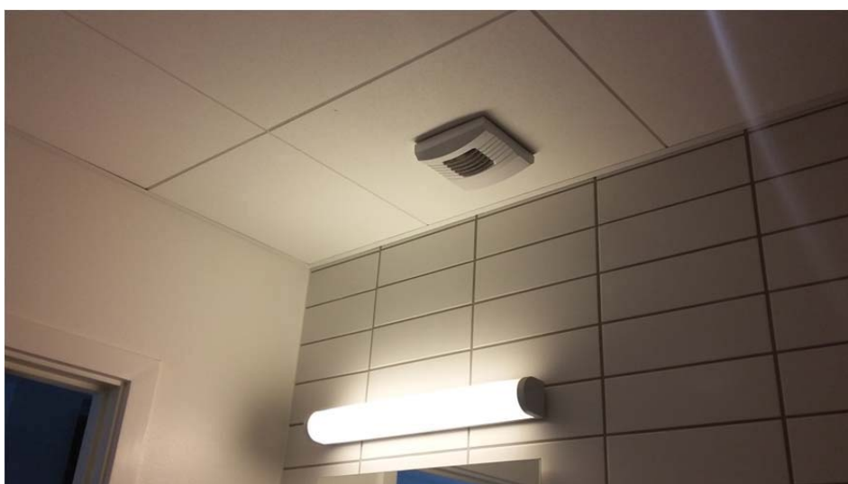
Air extract terminal, example
