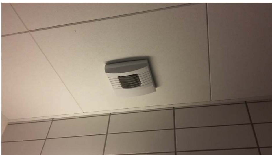
Air extract terminal, example
