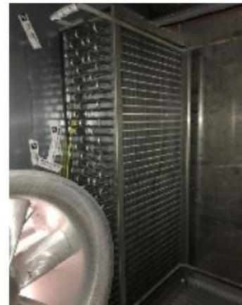
Figure 4: Evaporator coil and fan
