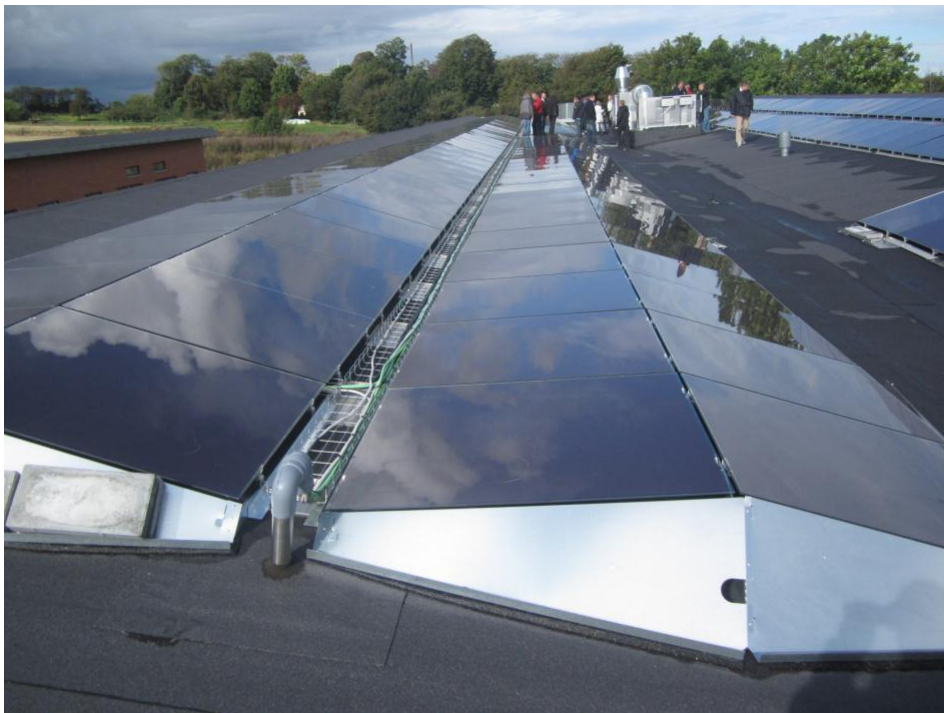
East-West installation with a-Si modules on the roof of Marienlyst old peoples home. Skive 18 September 2012
