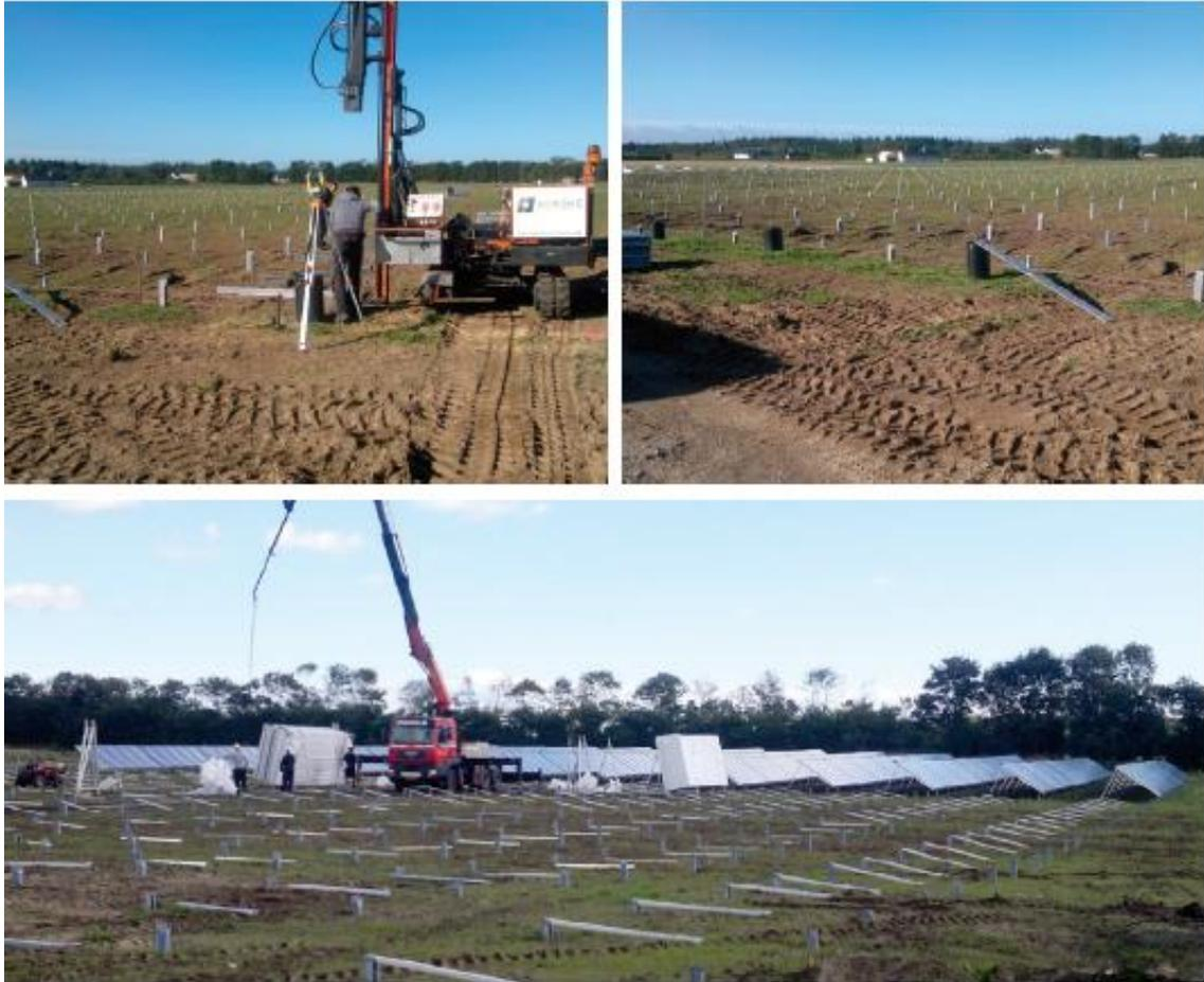
**Fig. 13:** Pictures from implementation of the solar collectors.
