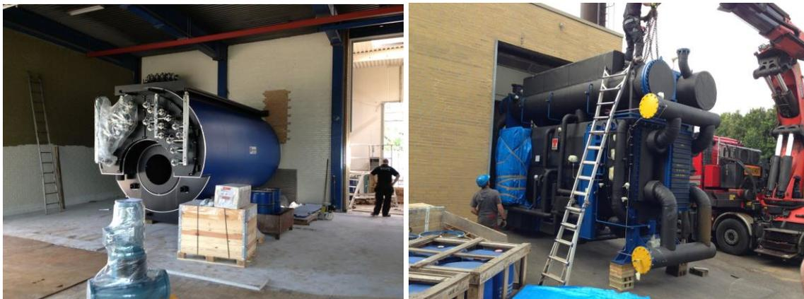
**Fig. 14:** Pictures from implementation in Søndervang (Boiler for absorption heat pump and absorption heat pump).
