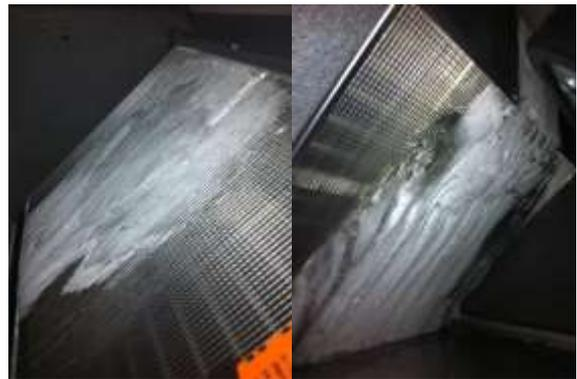
**Ice formation on air fins from EXHAUSTO A/S heat exchanger.**
