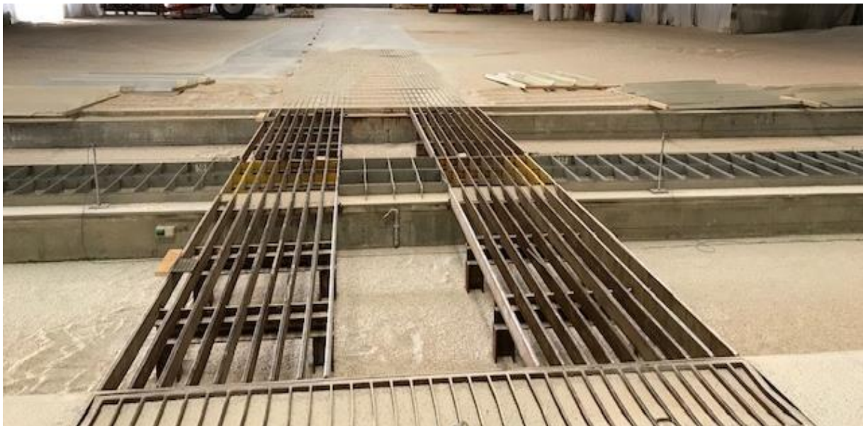
Figure 2. Bridge for driving across the measuring area consisting of 112 collectors in transverse direction
