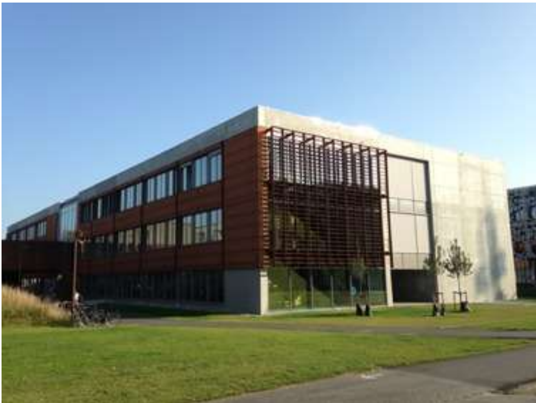
Figur 2.2. OU44 Building in Odense.
