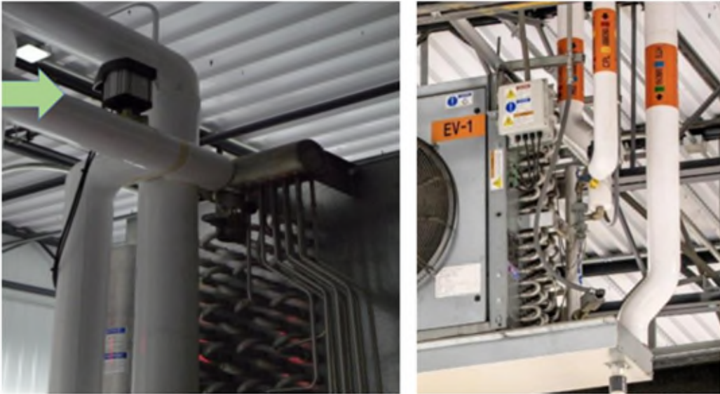
Figure 8: To the left a tank distributor and to the right a traditional distributor.
