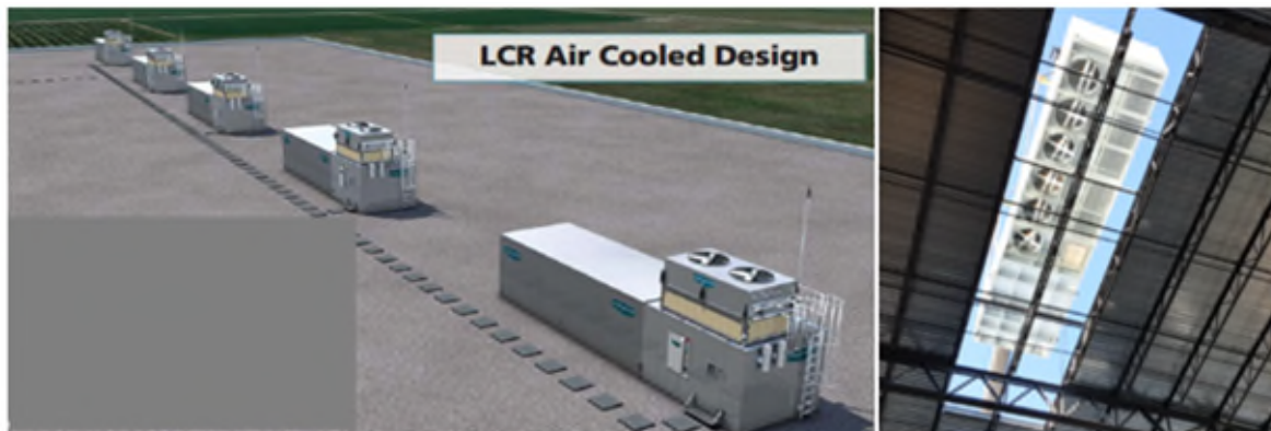
Figure 16: Evapcold air cooled unit placed on top of the building to the left, and unit lowered in place to the right.
