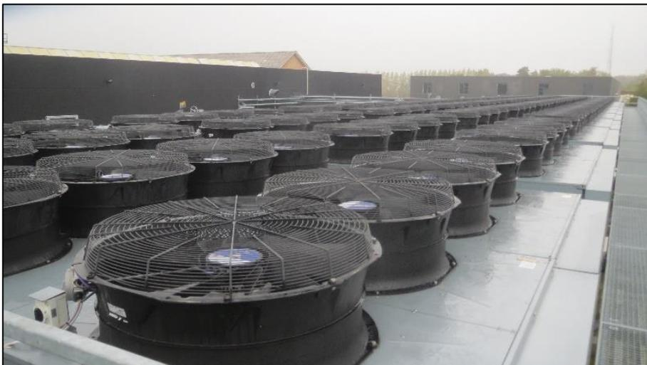
Figure 4: Picture of the evaporators at Brædstrup Fjernvarme
