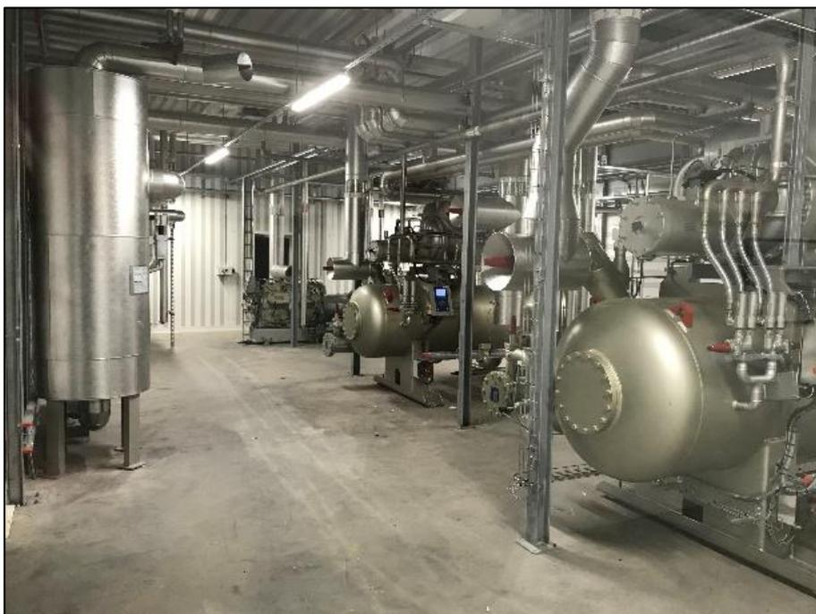
**Figure 1: Main components in the building for the heat pump**
