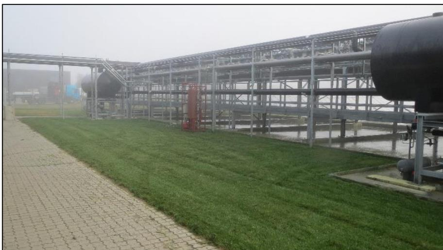
**Figure 2: Pump separators and evaporators placed outside**
