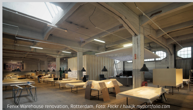
Fenix Warehouse renovation, Rotterdam. Foto: Flickr / haajik.myportfolio.com
