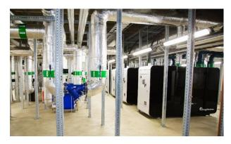
Figure 2: An Energy Machines installation. Heat pumps are located on the right. Sensors are placed inside the boxes.
