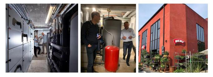
Figure 1: Heat is recovered from a supermarket refrigeration system to the local district heating grid in Nordhavn, Copenhagen.
