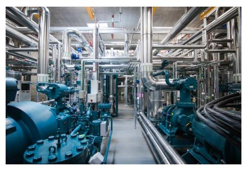
Figure 1: 5 MW<sub>thermal</sub> heat pump system for district heating in Copenhagen [Source: HOFOR].
