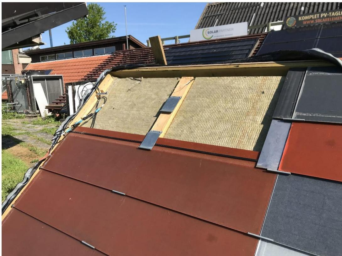
Figure 4: Photo of one of the mockups showing metal hooks and overlapping areas between the modules.
