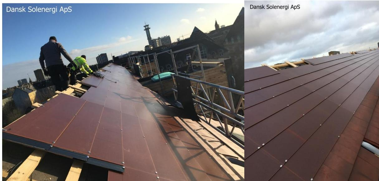
Figure 32 Renovation project with DSE modules in a flat tile roof construction
