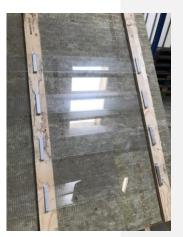
The PV elements are hung inside hooks that are in turn screwed to lattes. Installations of the PV panel are easier in this manner.
