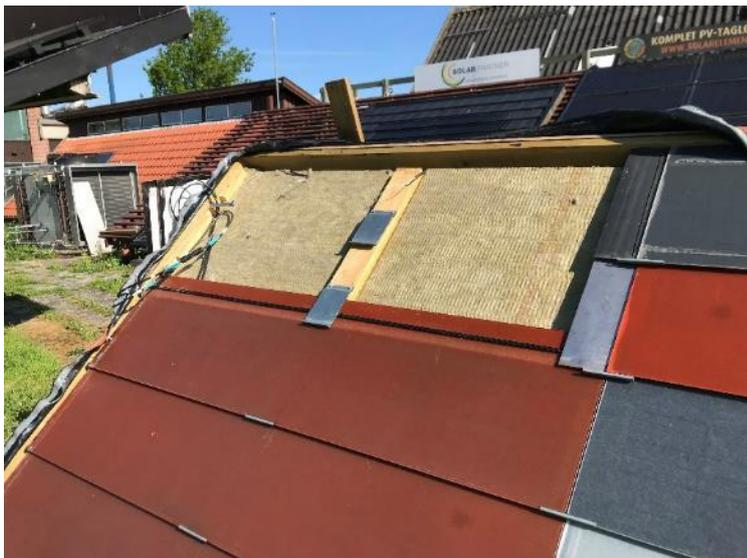
Figure 7 Removal of old modules from top and down. A rubber strip can be seen on the old module.
