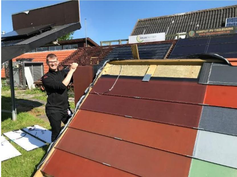
Figure 8 Two new modules mounted. There is no rubber strip on these.
