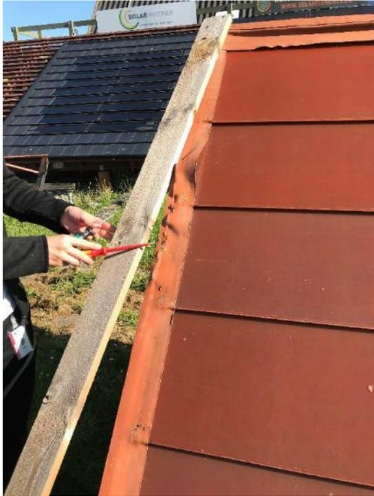
Figure 6 Disassembly of edge profile and bitumen tape.
