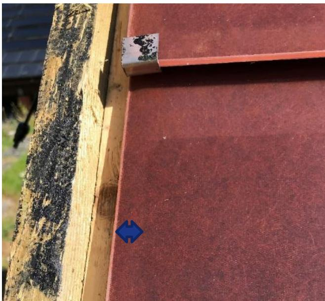
Figure 9 Due to narrow clearance from the PV cells to the edge of the glass, it was necessary to move the outer profile to avoid shadow of the cells.
