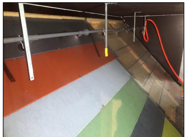
Photo 4 – Water spraying from nozzles
