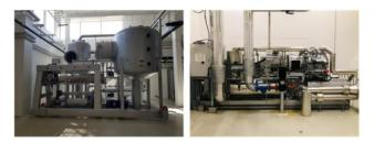
Figure 2 - Seawater and NH₃ heat pump system at Aarhus Ø (AVA) used for case study I.
