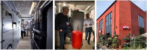
Figure 13. Heat is recovered from a supermarket refrigeration system to the local district heating grid in Copenhagen.
