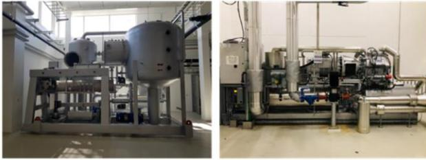
**Figure 2 - Seawater and NH<sub>3</sub> heat pump system at Aarhus Ø (AVA) used for case study I.**
