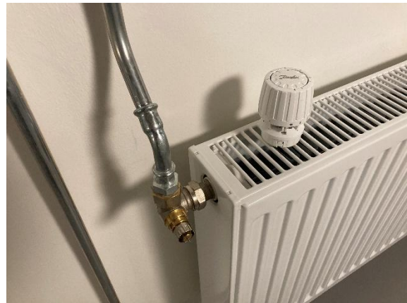
Figur 4.34 Forindstillelig manuel termostatventil
