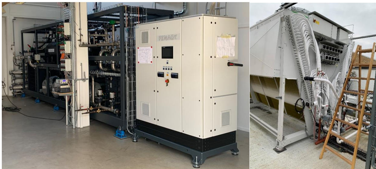
Figure 2: To the left is the heat pump that was developed in the project. To the right the reversible air source fin tube heat exchanger also developed in the project.
