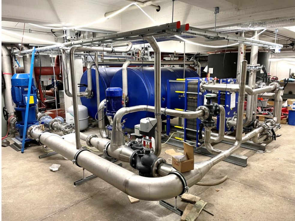
Figure 7: Part of the mixing loops built for the testing in the project.
